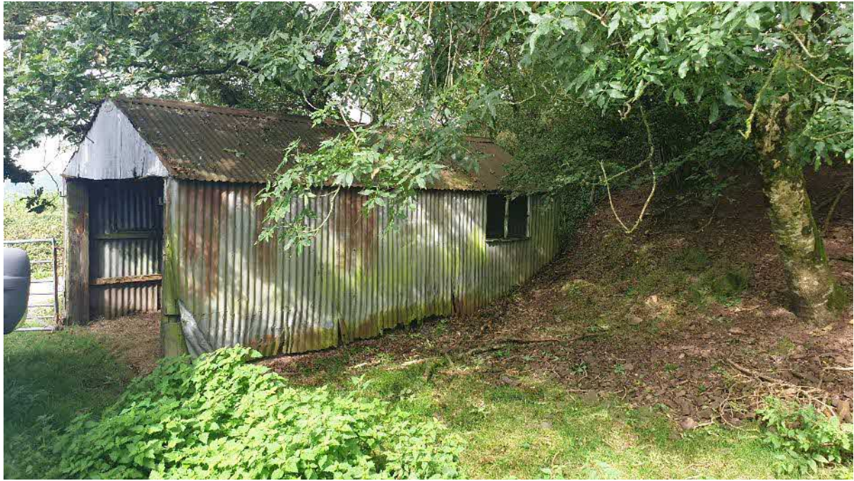
Photograph 6: Outbuilding 3 (outside of application site; to be retained)
