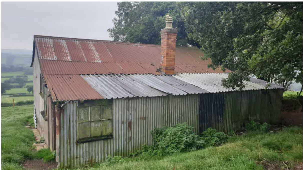
Photograph 2: Hele View from the rear (north)
