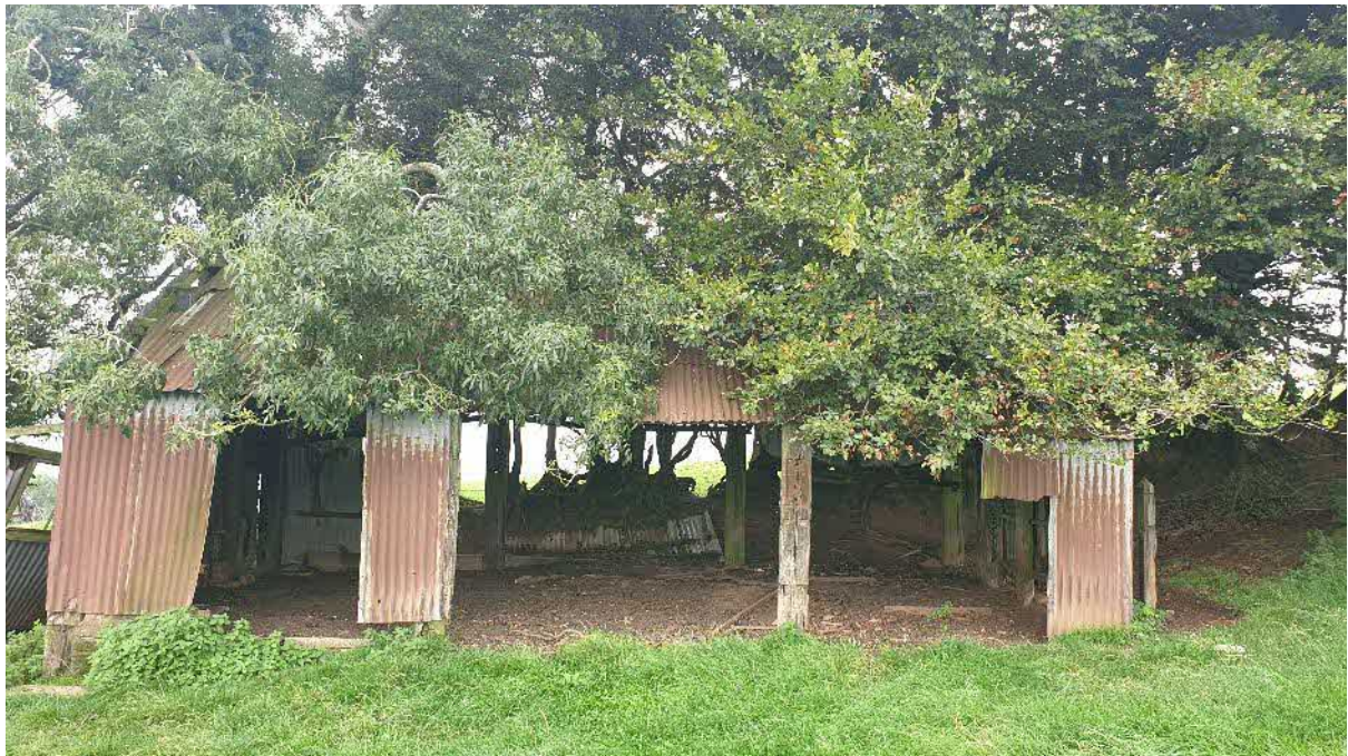
Photograph 5: Outbuilding 2 (to be converted into water storage/ancillary usage)
