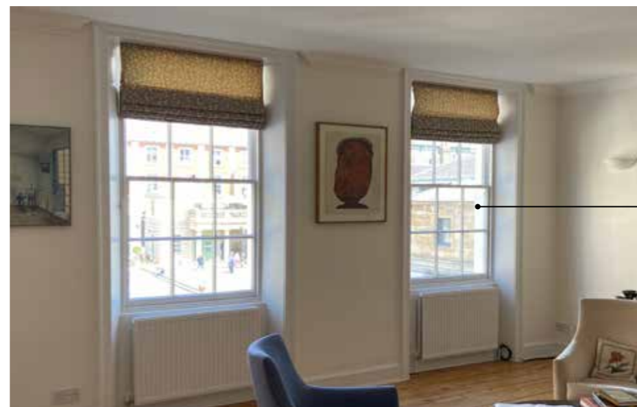
Existing windows internally, timber architraves to be retained
