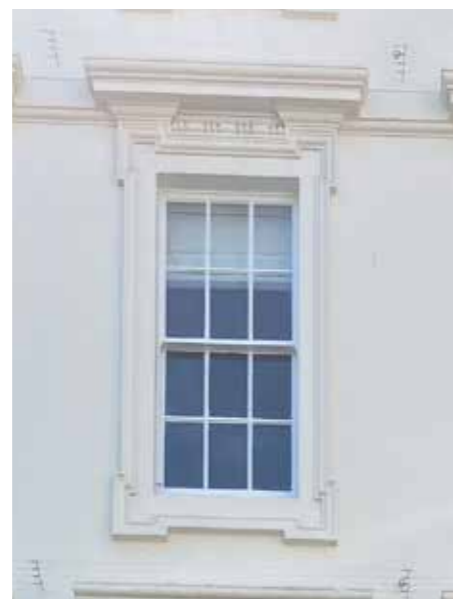
Existing window, external view
