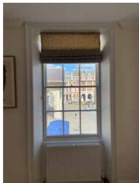
Existing window, internal view
