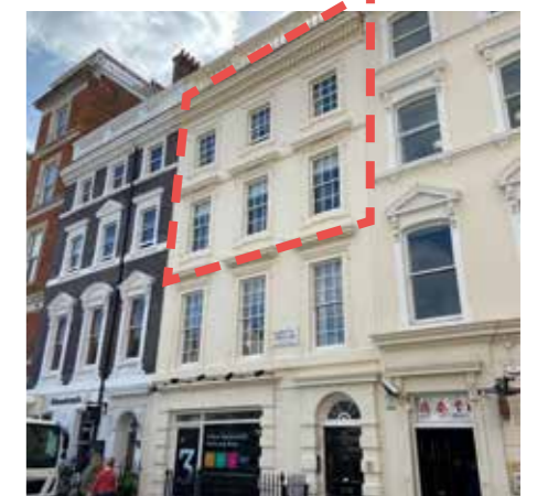
Contemporary photo showing windows with divided panes.
