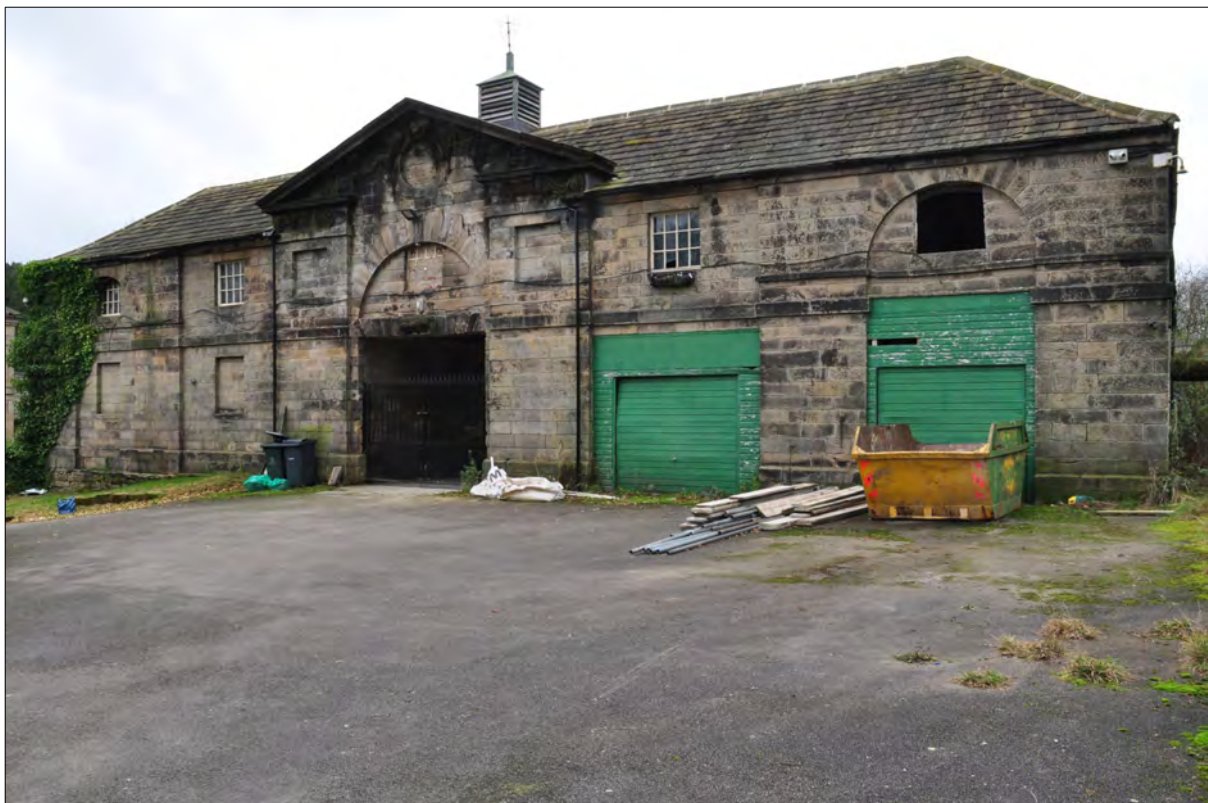
Photo 4: Front of east range
