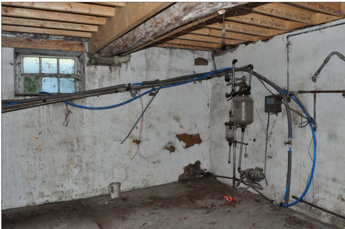
Photo 18: North range, ground floor, west end (room 4)
