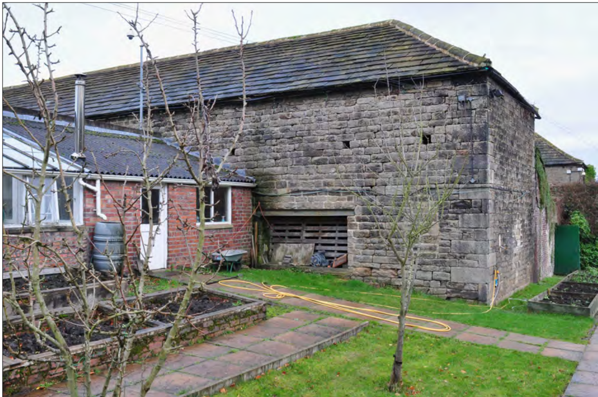
Photo 7: South end of west range
