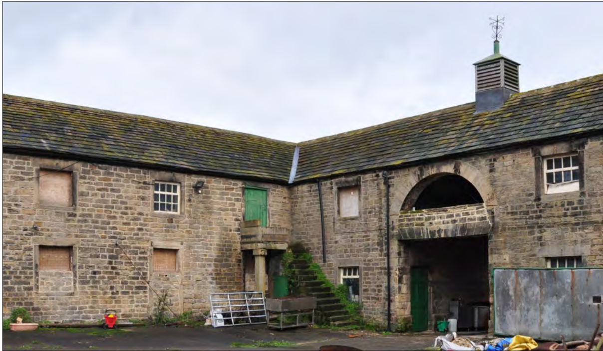
Photo 9: North-east corner of courtyard
