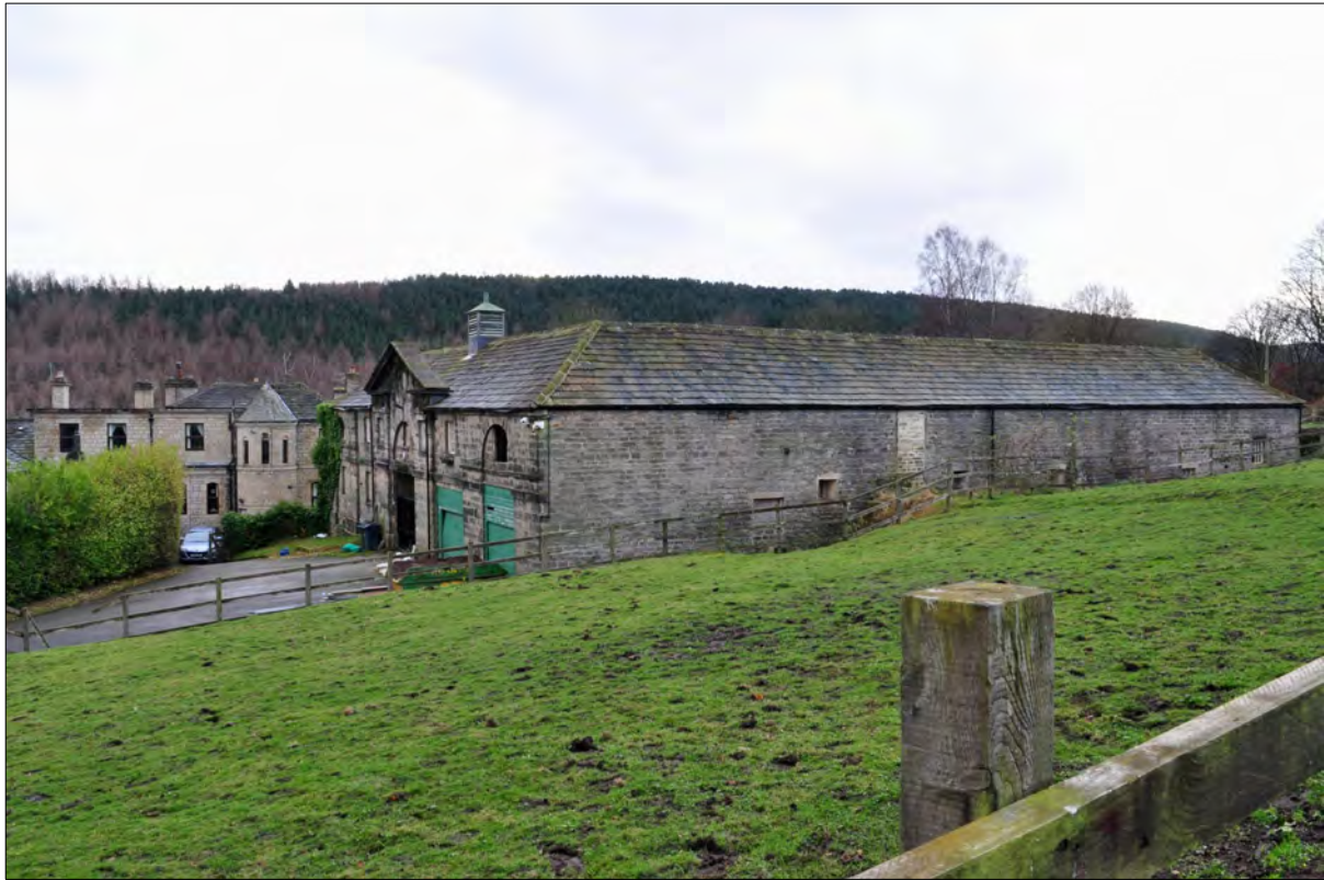
Photo 3: View from the north-east
