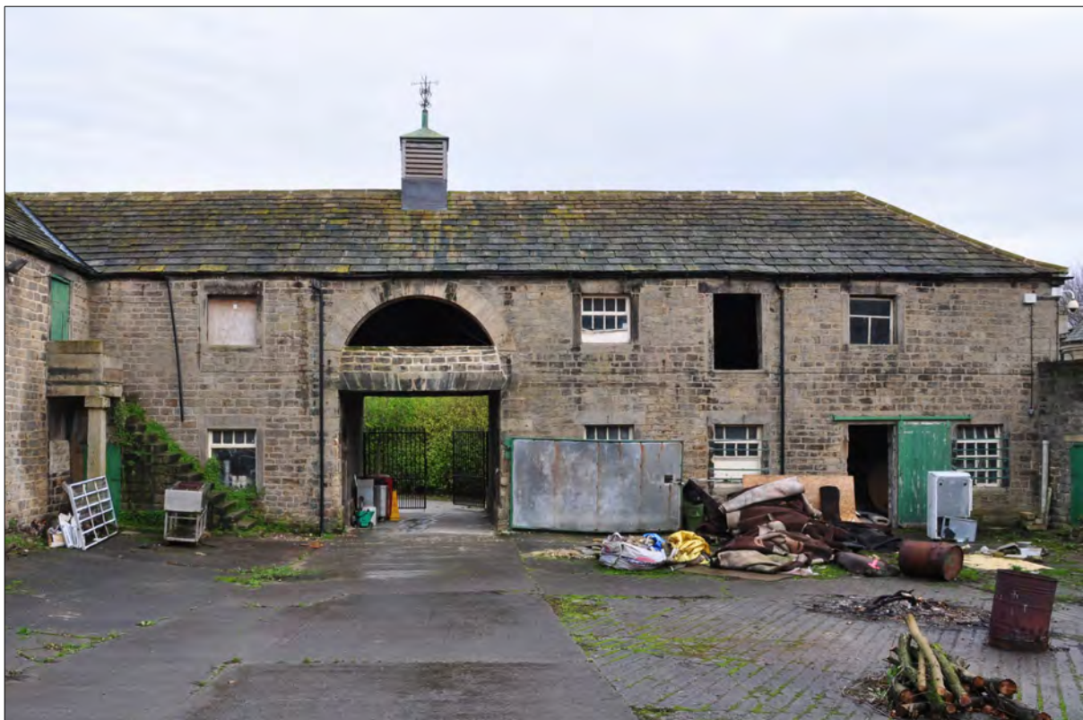
Photo 8: East range, facing onto courtyard
