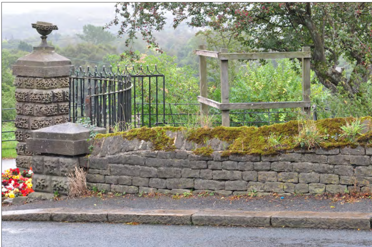
Photo 2: West side of gateway and boundary wall
