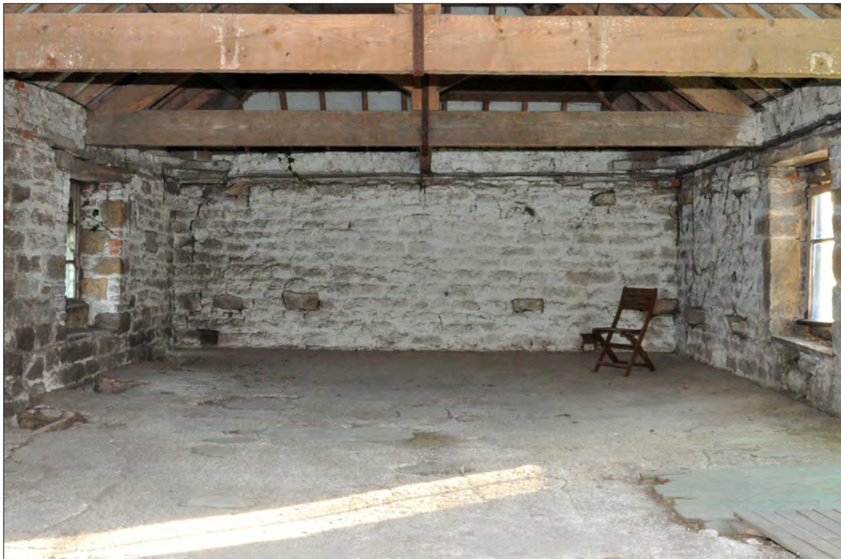
Photo 17: First floor, east range, south end (room 9)
