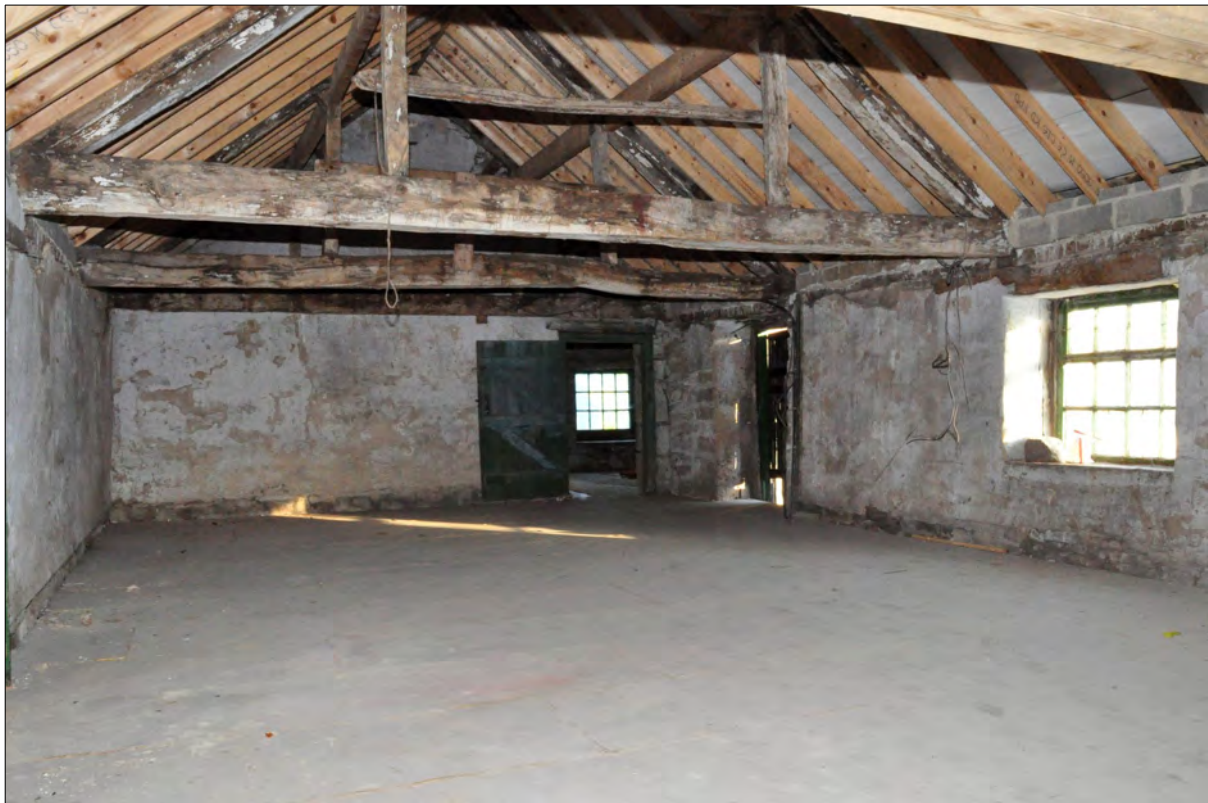
Photo 19: North range, first floor, east end (room 12)
