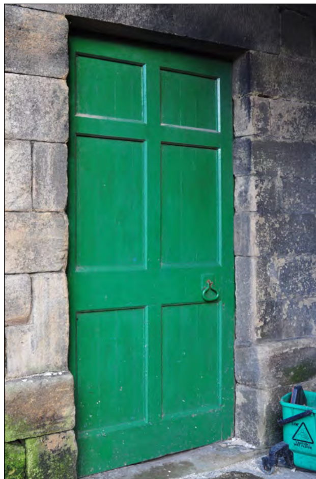
Photo 10: One of two historic doors off covered entry, east range
