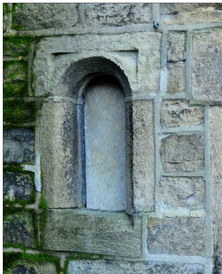
Photo 12: Re-used 17th century window, north range
