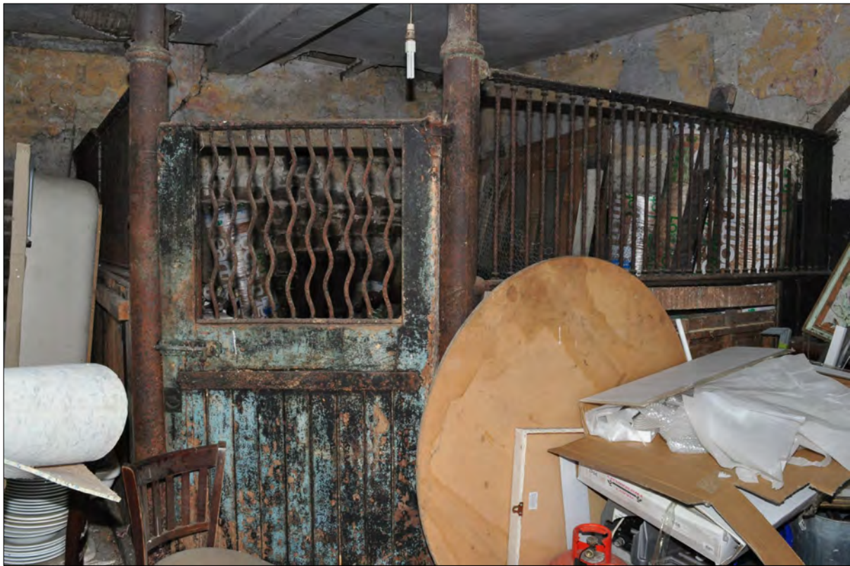
Photo 15: Non-original stable fittings, east range, south room (room 2)
