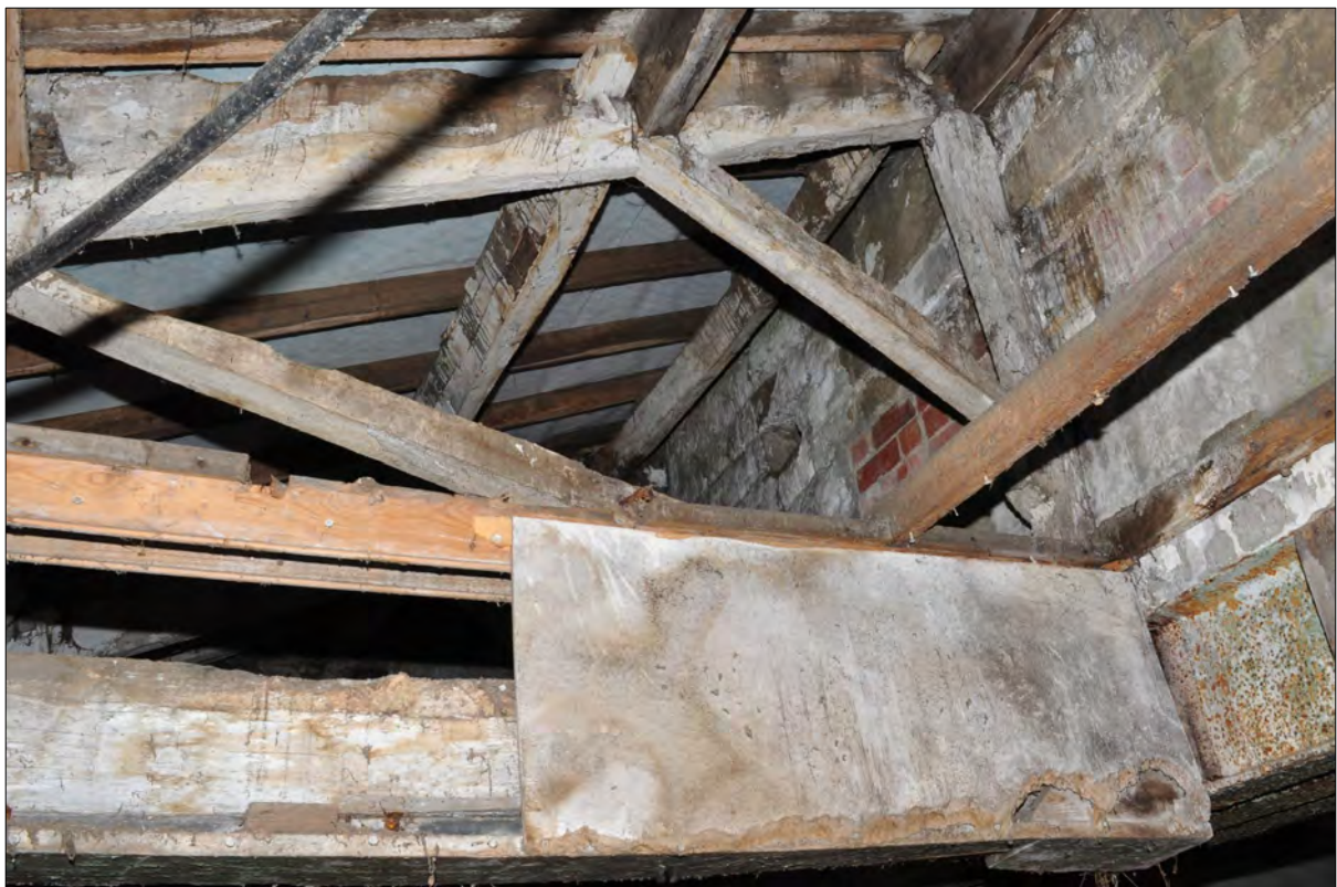
Photo 22: Outshut to west range: original roof structure
