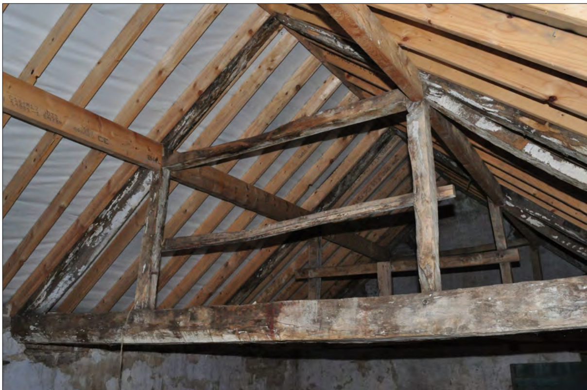
Photo 20: North range: original roof truss (room 12)
