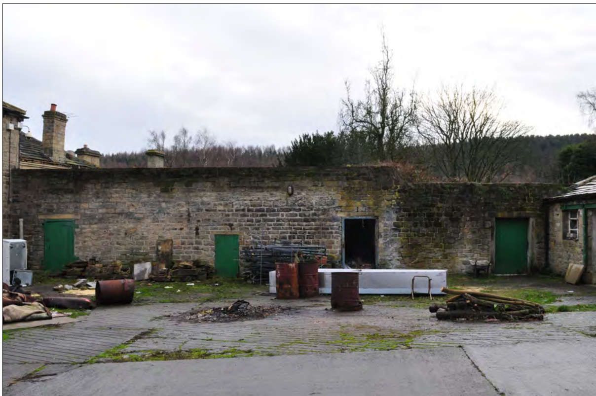
Photo 14: Rear of garden wall forming south side of courtyard
