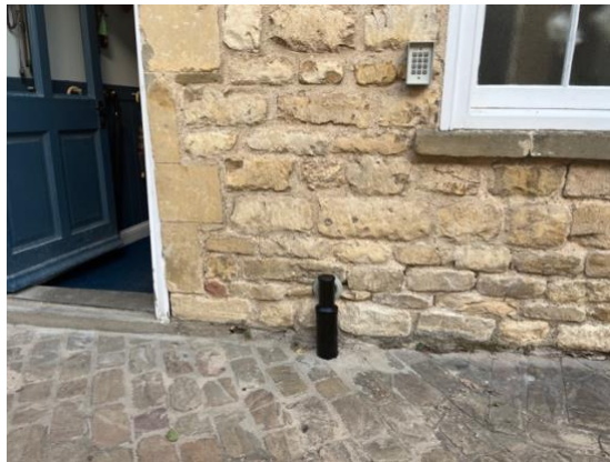
Above: The installed pipe to internal meter
