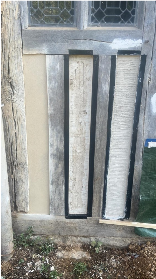
Fig. 5 (left): Sample panels showing stages of three-coat work with finished (unpigmented) panel on the left hand side.
