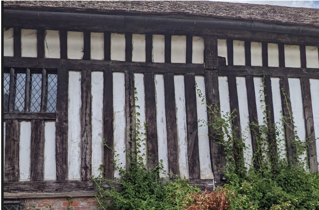
Fig 3. (above) Upper part of the east elevation of the north courtyard. The late C20 restoration was not completed and it is clear that this section was left until last and not repaired. The infill is clearly cement Based and will need to be removed and replaced with lime render.
