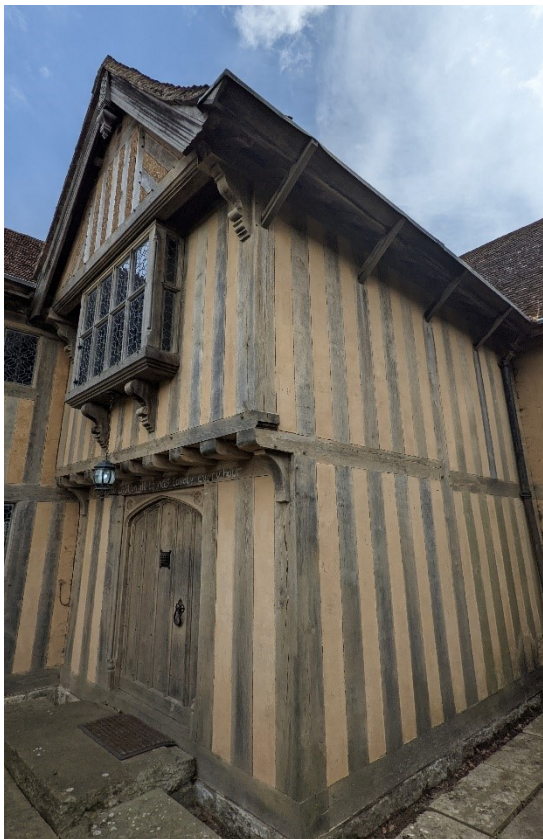
Fig 3. (above) Upper part of the east elevation of the north courtyard. The late C20 restoration was not completed and it is clear that this section was left until last and not repaired. The infill is clearly cement Based and will need to be removed and replaced with lime render.
