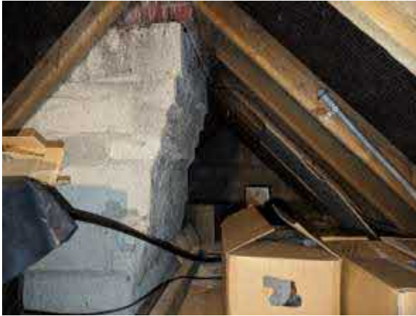
Photo 3. Showing the roof void over the house below the ridge
