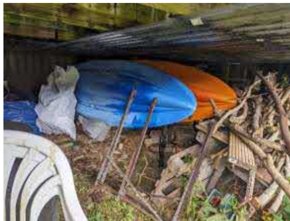
Photo 5. Showing the area below the decking
