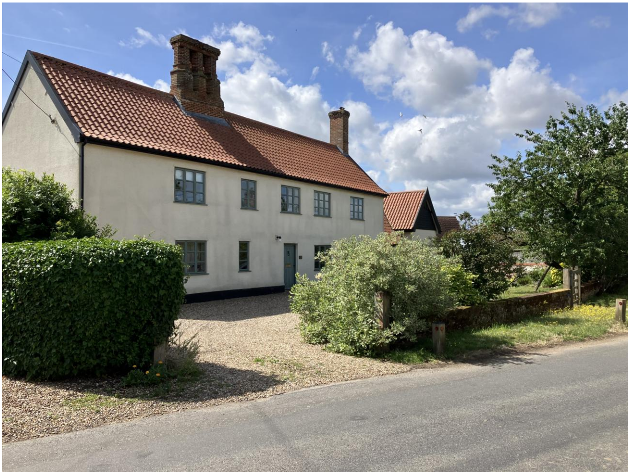
Photograph of the Existing Front Elevation
