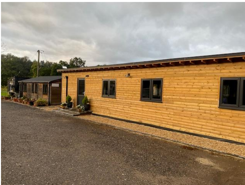
Photo.1 – Front elevations of former office space in the foreground and new office building beyond
