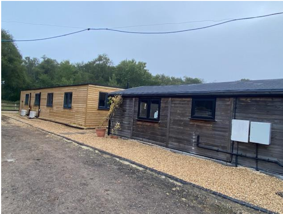
Photo.2 – Rear elevations of new and old office buildings
