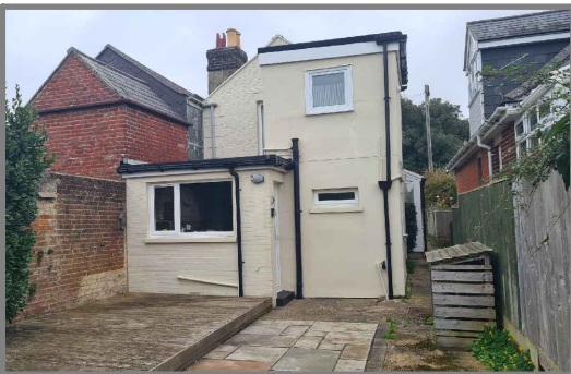
[REAR OF PROPERTY - 35 WORSLEY ROAD]
