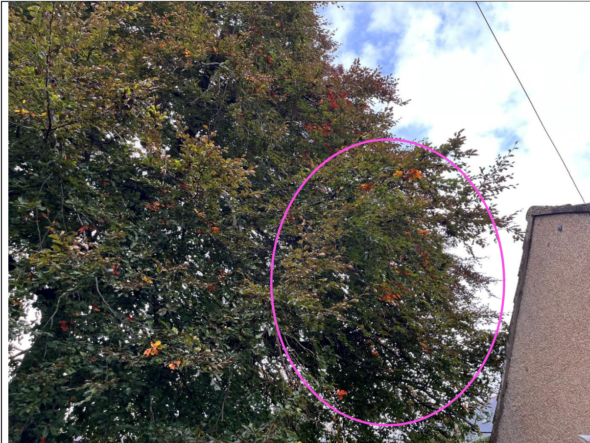
9. Section of the crown to be pruned back 3m from number 43
