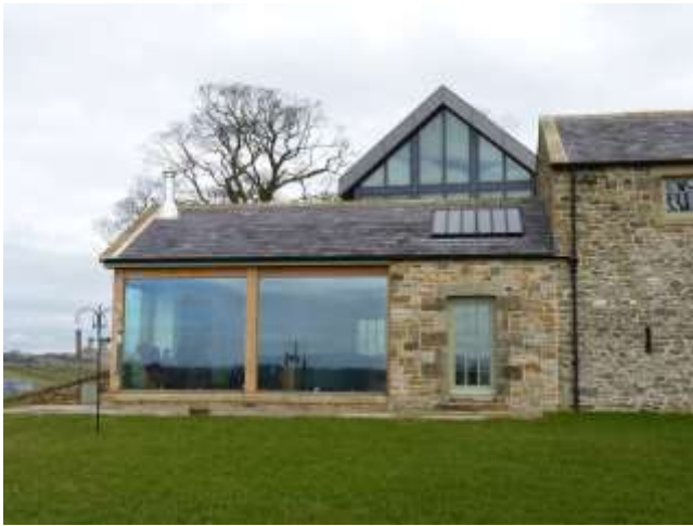
Left: Example of barn conversion with new large south westerly openings, Northumberland (Scheduled Monument, Listed Building, National Park and World Heritage Site)
