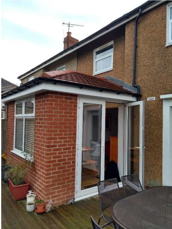
Existing Pitch-Roofed, Brick-Facing Extension
