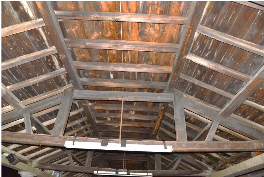
The existing roof soffit
