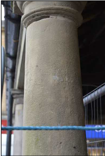
COLUMN Original Hit by car Realign Large indent required at base
