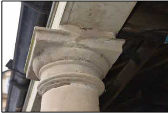
HEAD Original NHL plastic repair to top rib Realign
