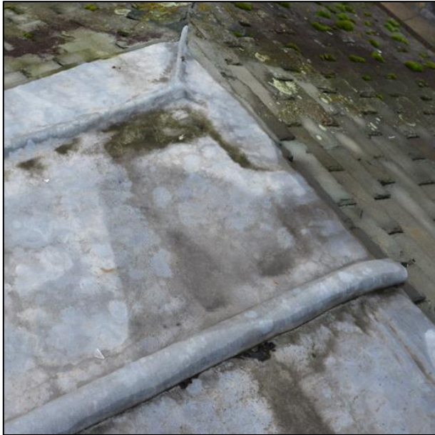
The east and west end panels of lead have welded lead mitres at the corners, and they are fixed down using copper nails into the side of the final rolls.
