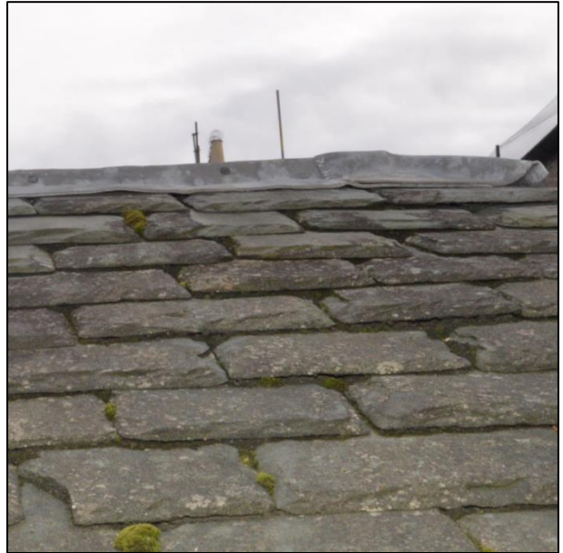
The east and west end panels of lead have welded lead mitres at the corners, and they are fixed down using copper nails into the side of the final rolls.
