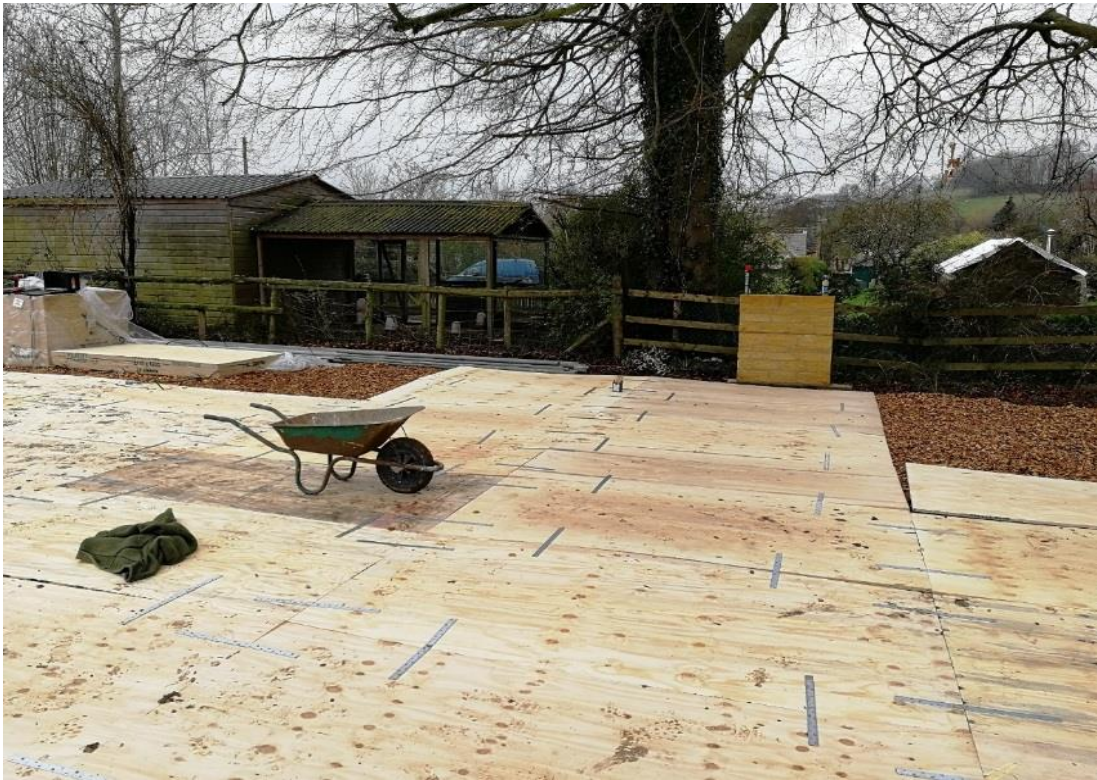
Figure 6 – Plywood sheeting used as ground protection.
