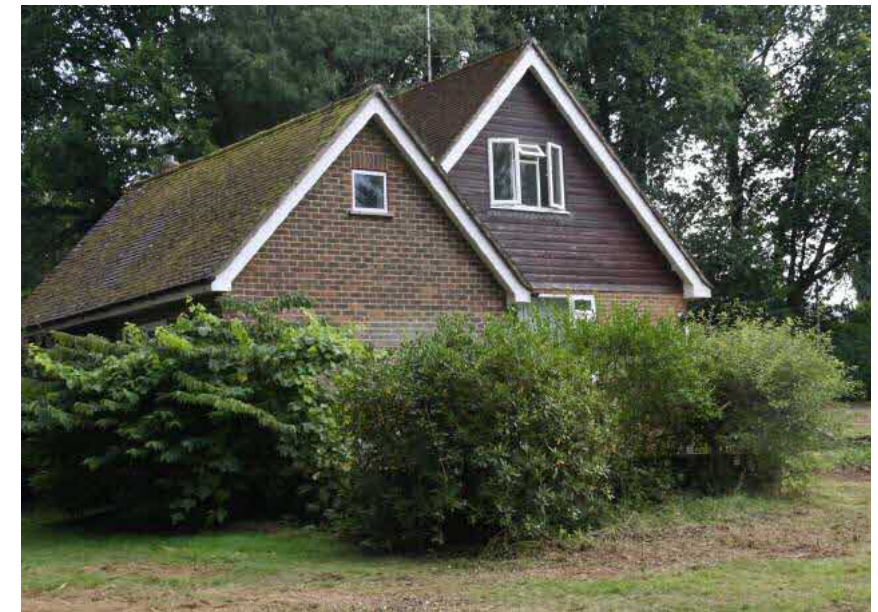
2. View of West facing elevation
