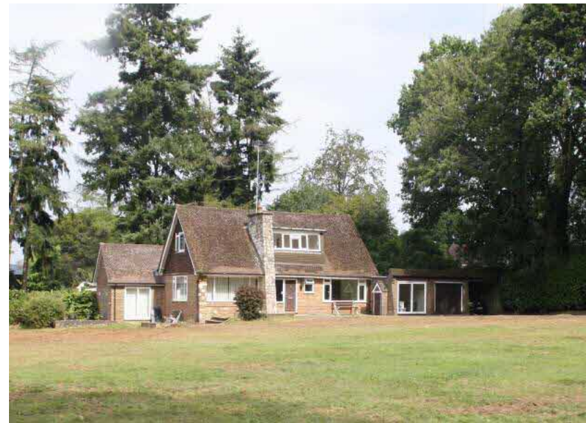
1. View of south facing elevation
