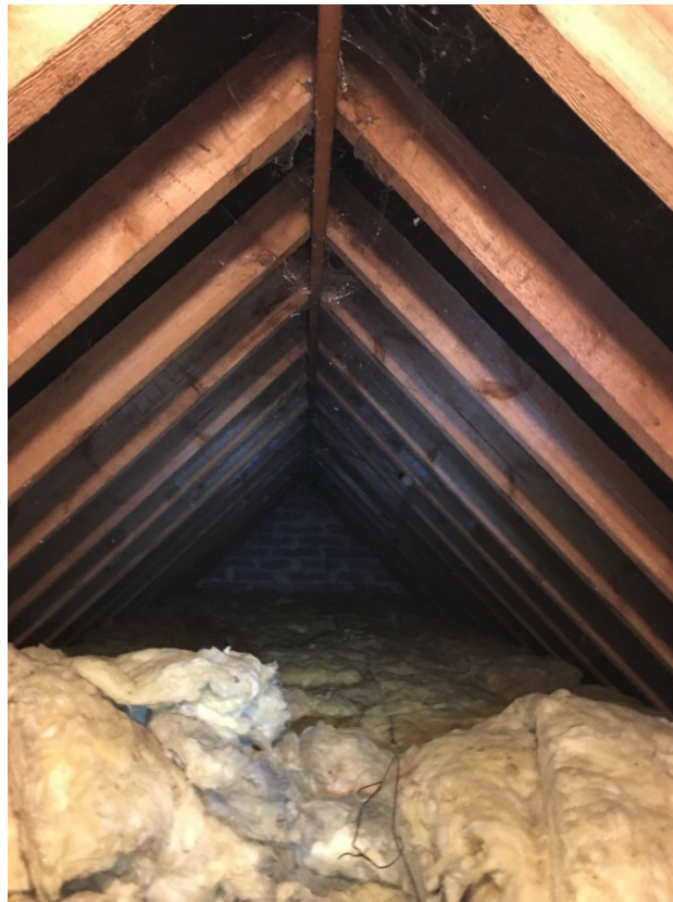
Figure 8. Loft void looking east.
