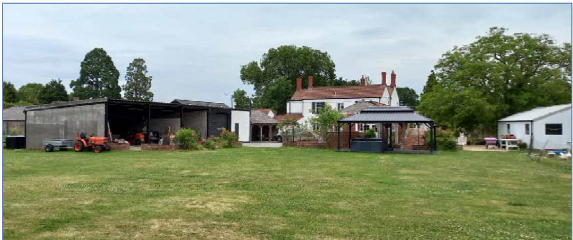
Fig 3. Photograph of the ancillary building proposed for development in situ with the main property.
