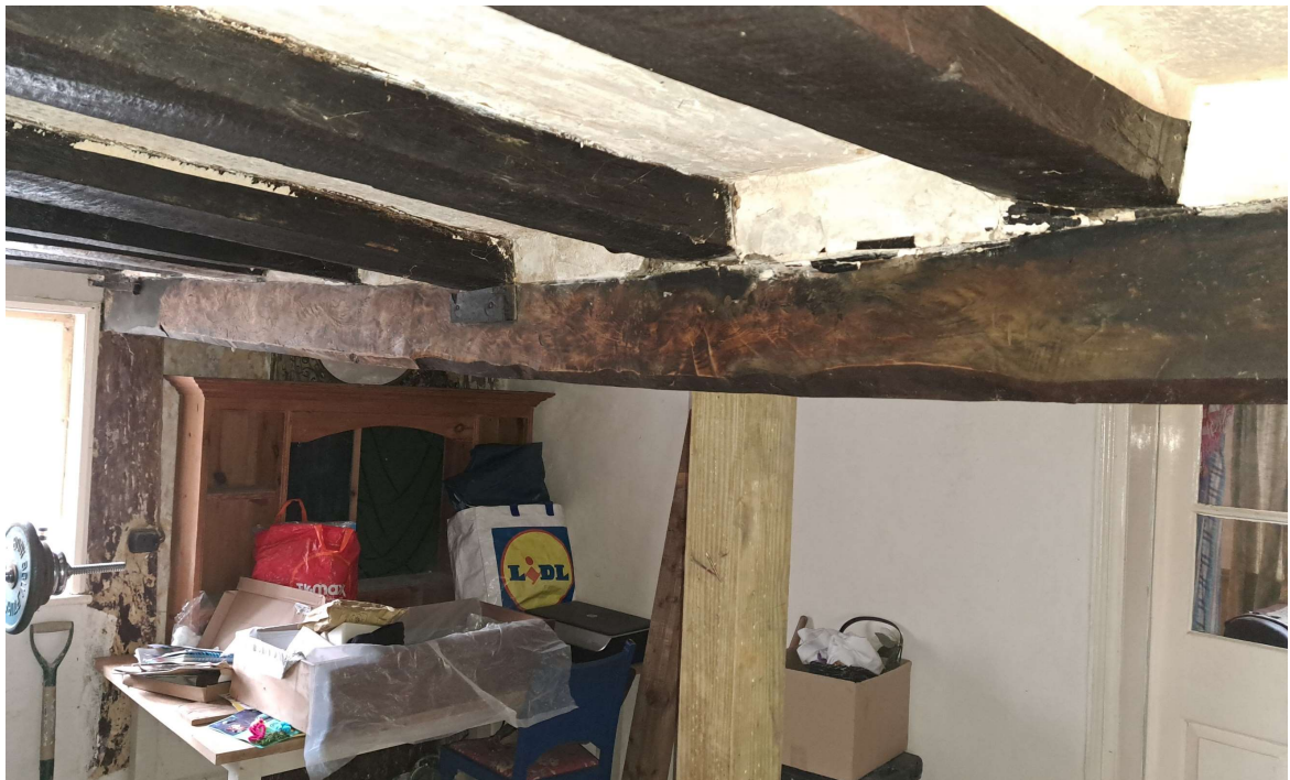
Figure 8 Propped Beam
