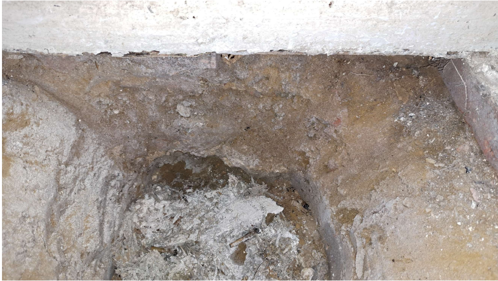
Figure 9 Trial Pit - No Foundations
