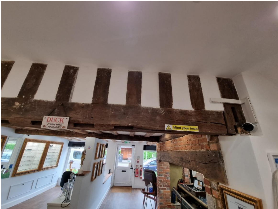
Figure 4 – view from rear of shop towards front elevation.
