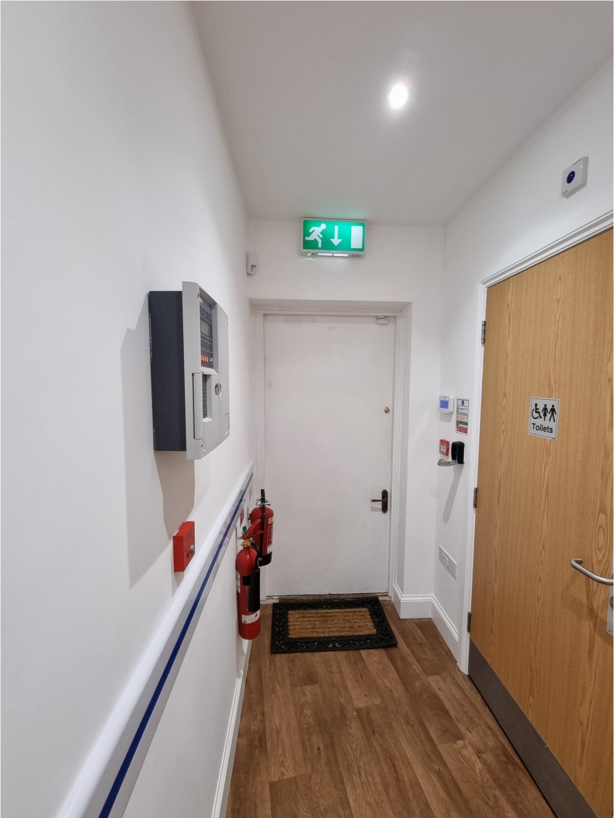
Figure 2 - new partitions inserted into rear extension.
