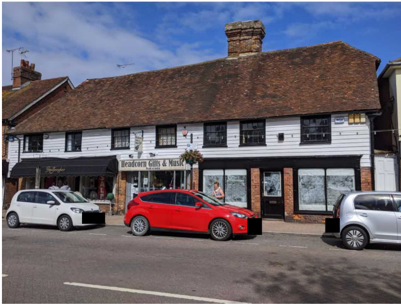
Figure 1: Main front elevation of the subject site, facing onto High Street
