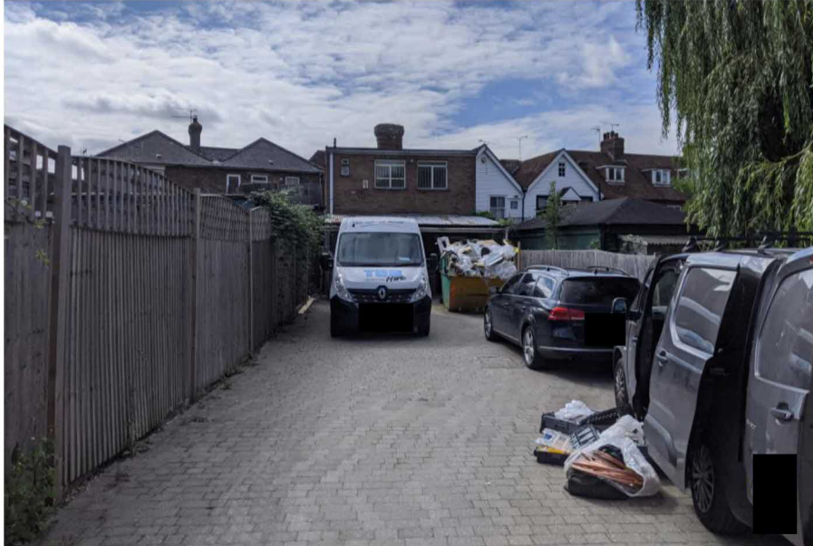
Figure 3: Rear elevation of the site. There is a long driveway with the 1970s extension to the rear. The original part of the listed building is mostly concealed.
