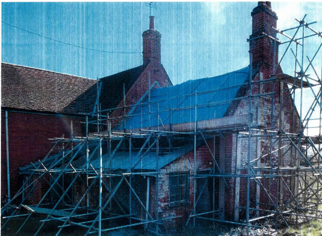
Temporary Scaffolding Installed Around Cottage (View from North/Rear)
