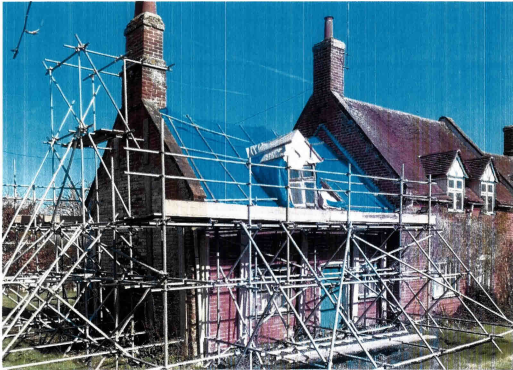
Temporary Scaffolding Installed Around Cottage (View from South/Front)
