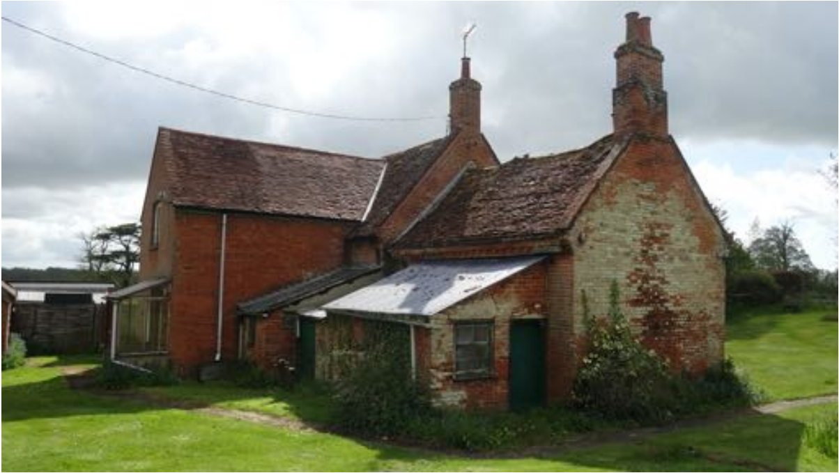
Image 4. West Elevation (May 2021). This images shows both 23 & 24 with the single storey lean-to additional and the two storey extension to the rear of no. 24.
