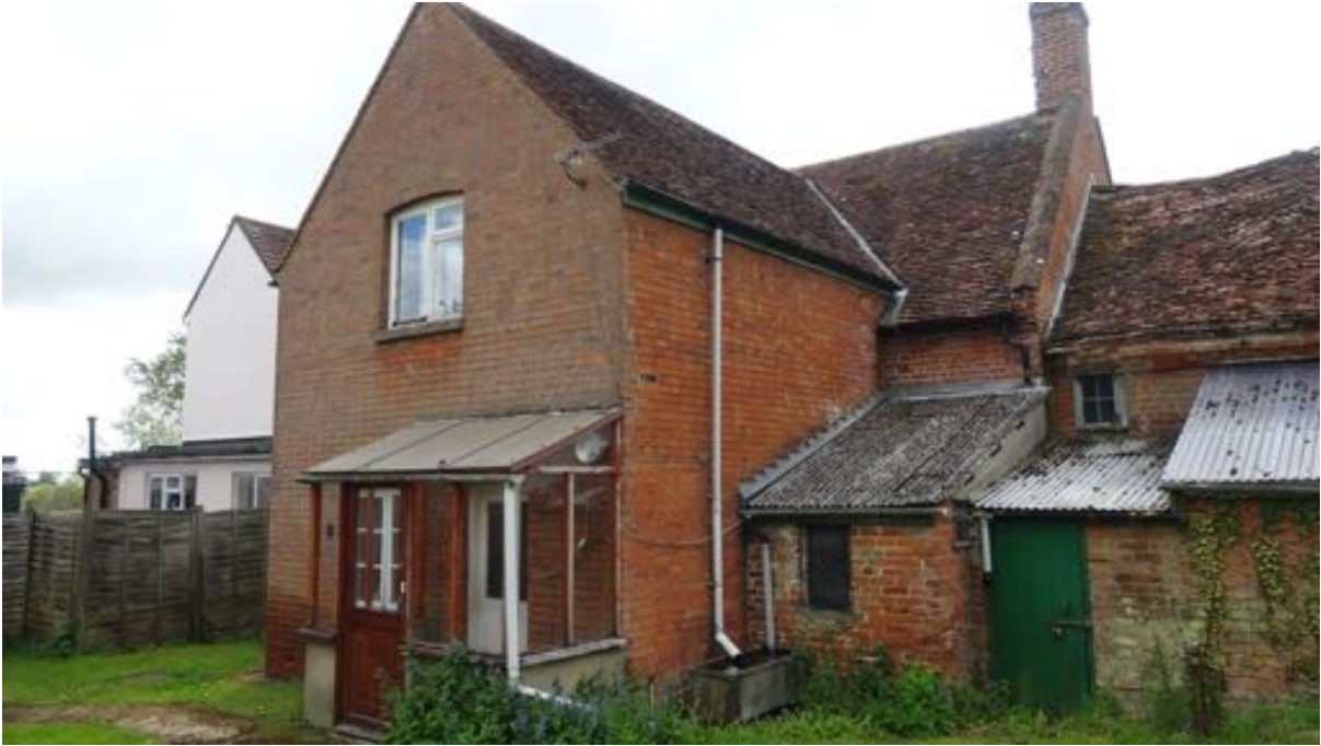
Image 6. North Elevation (May 2021). This shows the latter addition 2 storey rear extension to the rear of no. 23 along with the single storey lean-to additions to the rear of both 23 & 24.
