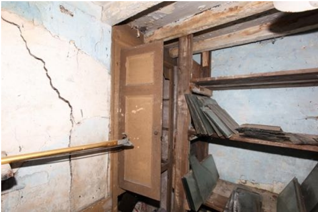
Illus. 20. The 19 th century panelled doors of the cupboard to the north of the western fireplace in the sitting room at no. 24 (G1). Like the other doors of the room they retain what appears to be their original paintwork.
