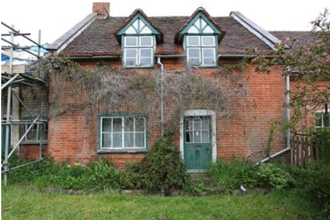
Illus. 6. The projecting or 'breakfront' southern facade of no. 23 showing the Mock Tudor dormer windows that probably date from the later refurbishment of circa 1910 that included the rear extension. The brickwork is identical to that of Lodge Cottage on the right but the flat tops of the brick arches above the ground-floor window and entrance door differ from their arched counterparts at no. 24.
