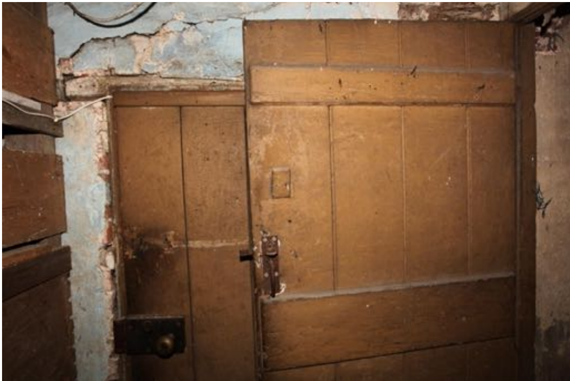
Illus. 22. A detail of the plank-and-batten stair door in the north-eastern corner of the sitting room at no. 24 with the door to the lean-to 'garden room' on the left (G1). Both retain original or early paintwork and an original wooden pull handle is visible above the latch of the stair door.
