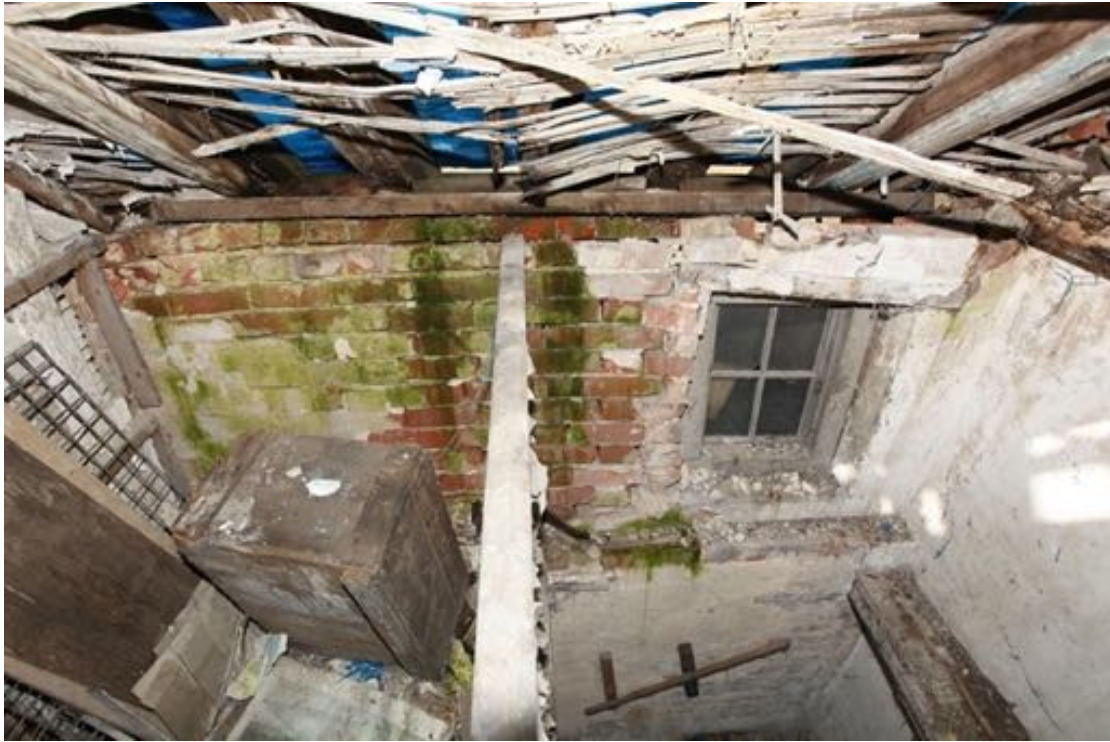
Illus. 27. The first-floor stair landing in no. 24 showing its window in the northern wall and the boarded partition framing the stair trap (F2).
