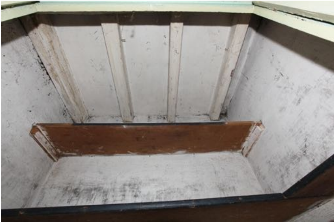
Illus. 39. The ceiling joists exposed in the cupboard shown in illustration 38 (G5). Their small chamfers and lack of lath nails indicate they were intended to be exposed like those in no. 24 and presumably extend to the rest of the sitting room where they are now concealed by later plaster.
