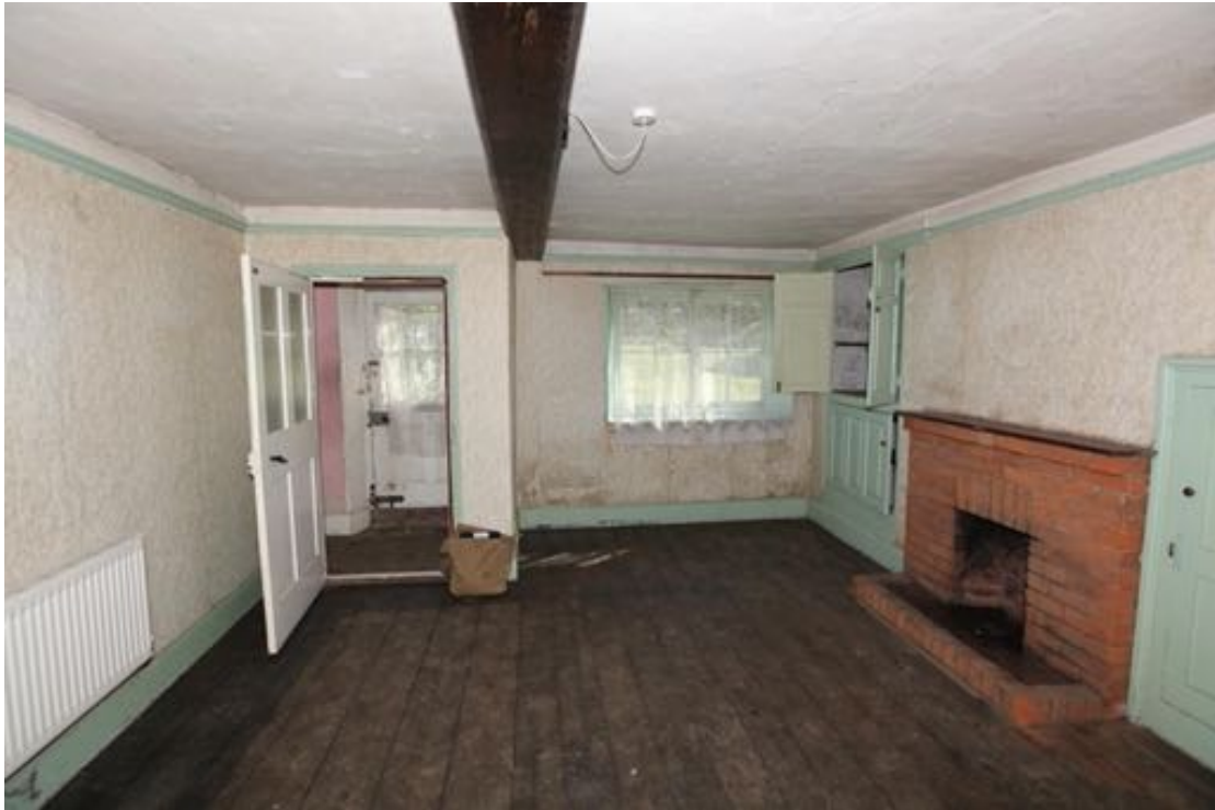
Illus. 43. The front (southern) interior of the sitting room at no. 23 showing its internal porch, horizontally sliding sash window and wide deal floorboards (G5).
