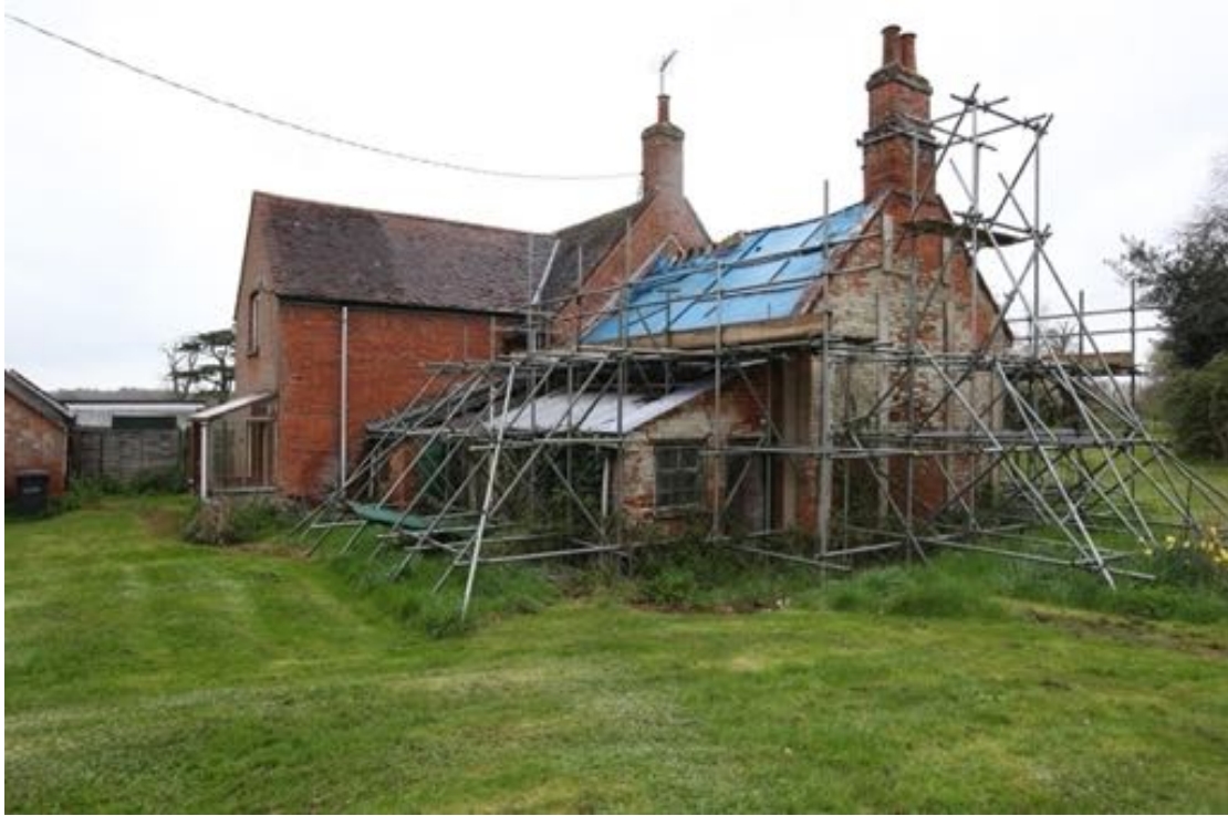
Illus. 7. The building from the north-west showing the brick lean-to 'garden room' behind no. 24 in the foreground and the two-storied rear extension of no. 23 added between 1902 and 1924. The 19 th century brick shed on the left contains a small chimney and was probably a wash house for no. 23 shared with Lodge Cottage.
