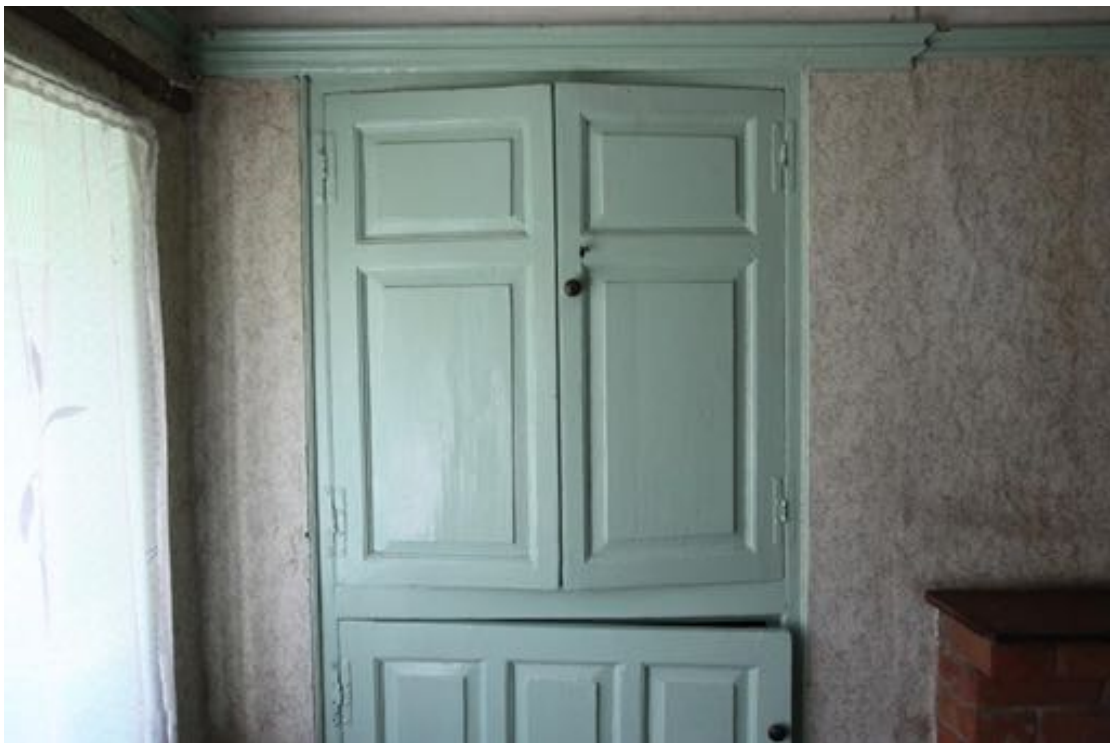
Illus. 38. A detail of the early- to mid-19 th century cupboard doors with fielded panels to the left of the fireplace in illustration 37 showing their Georgian H-hinges (G5). The plain panelled cupboard door to the right of the fireplace is a late-19 th century insertion with rectangular butterfly hinges.
