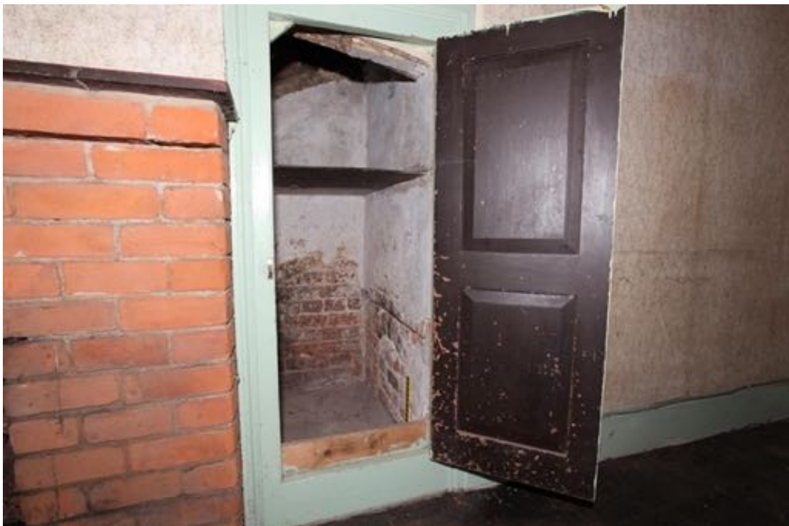
Illus. 40. The cupboard door to the right of the fireplace in illustration 37 opened to reveal its 19 th century brown paint and the side of the wider original fireplace with evidence of a bread oven (illustration 41).
