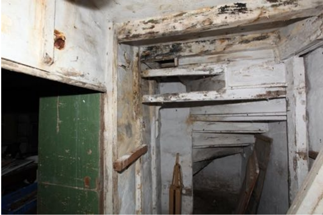
Illus. 25. The storage area in front of the stair at no. 24 (G2), as seen from the south with the partition adjoining the sitting room on the left. The shaped bracket of a missing shelf is nailed to a stud of the partition.
