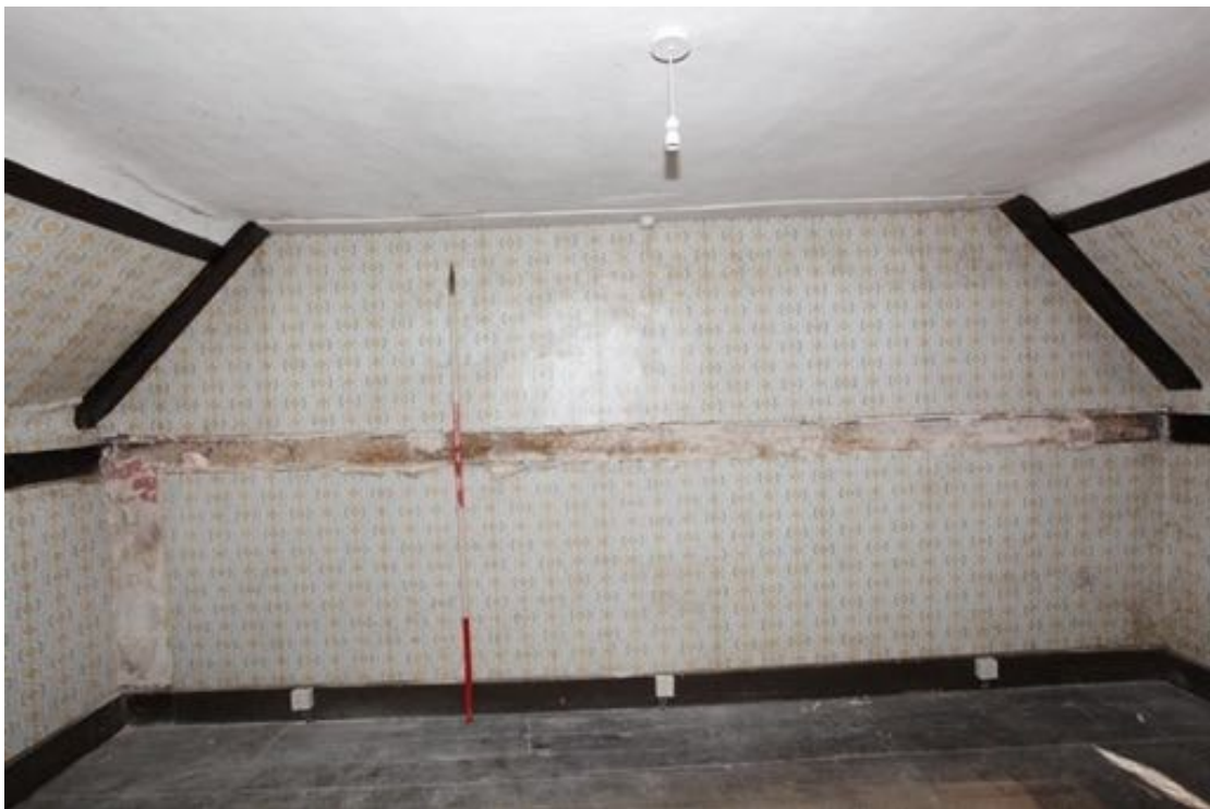
Illus. 48. The eastern internal gable of the eastern bedroom in no. 23 (F4) showing the lower of the two tiers of staggered butt-purlins and a tie-beam that is notched over the narrower walls of Lodge Cottage (illustration 49).
