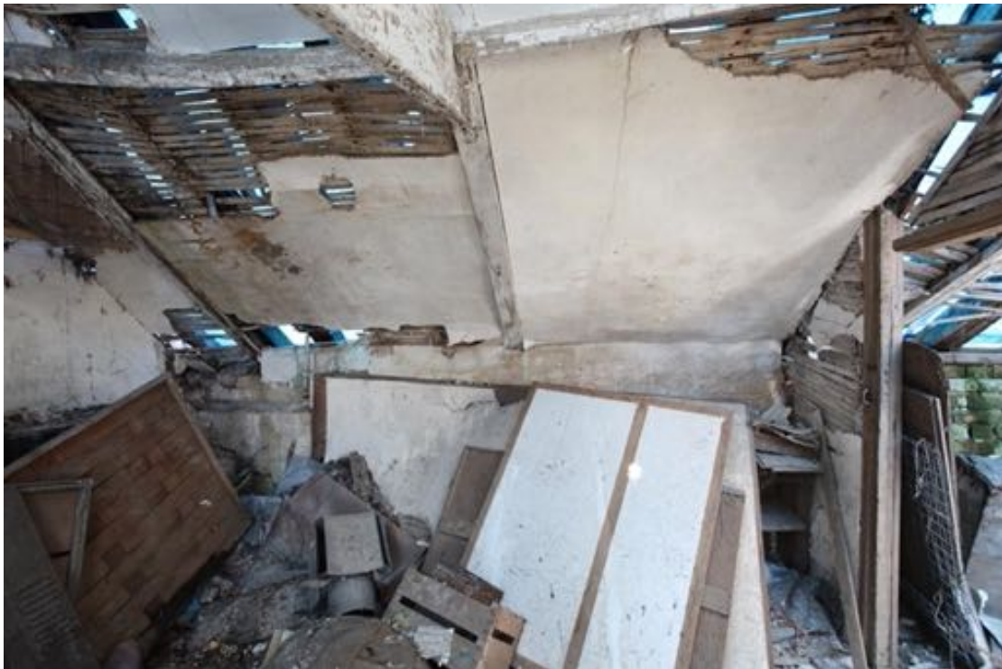
Illus. 36. The northern internal wall of the first-floor bedroom at no 24 showing its lack of windows and the structure of its clasped-purlin roof (F1).
