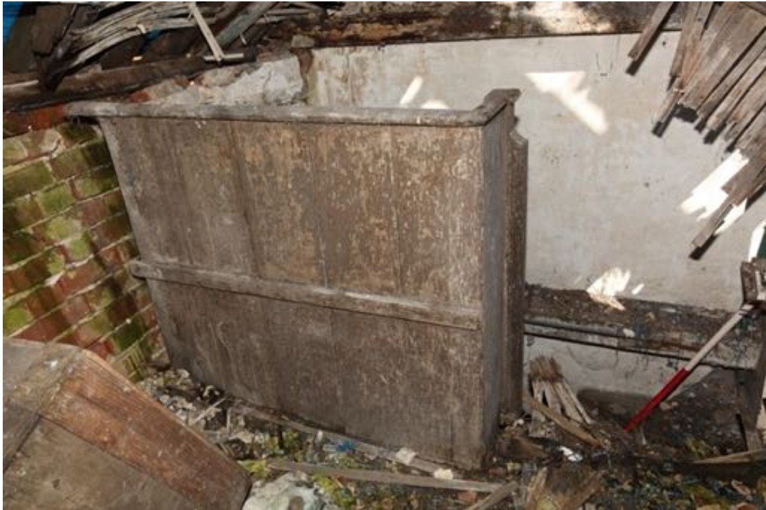
Illus. 31. A detail from the west of the 19 th century plank-and-batten partition adjoining the corner stair of no. 24 showing its original or early brown paintwork with the exposed 19 th century brickwork of the northern wall on the left (F2).
