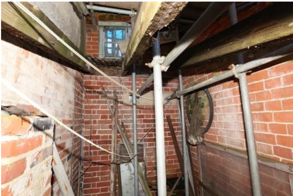
Illus. 10. The rear wall of no. 24 from the narrow gap between its rear lean-to and that of no. 23 on the left (G4). The corner of the brickwork is respected by closers on the left and is not integral with the fabric of no. 23 which projects by approximately 0.4 m to the north just as it does to the south. The stair window above is respected by the bonding.
