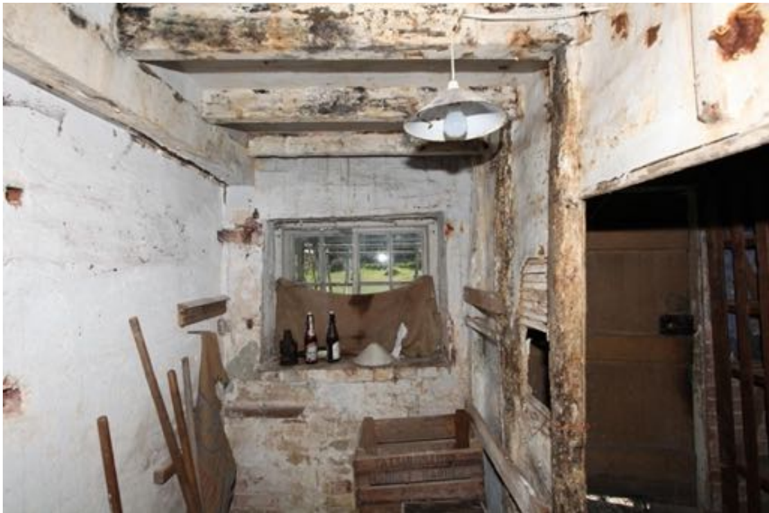
Illus. 24. The storage area in front of the staircase (G2) with the lath-and-plaster partition adjoining the sitting room of no. 24 on the right. This area may have been unlit initially as the horizontal sash window lies beneath a segmental arch that differs from the others of the southern facade and appears to be an insertion.
