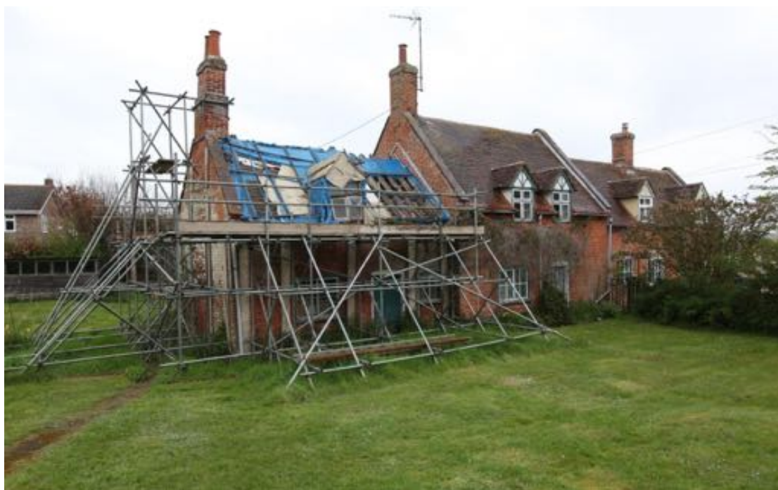
Illus. 1. The three cottages from the south-west, with the semi-derelict no. 24 on the left, no. 23 projecting in the centre and Lodge Cottage in separate ownership to the right. Lodge Cottage was not inspected for the purpose of this report, but the brickwork of its facade is identical to that of no. 23 and contains evidence of a vertical junction indicating the section to the right of its chimney was added later.
