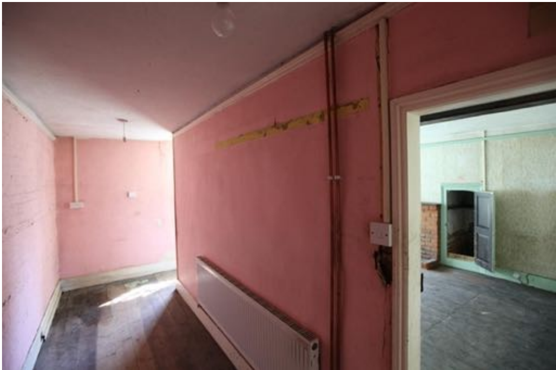
Illus. 44. The entrance passage to the east of no. 23 as seen from the rear (north) with the door to the sitting room on the right (G6). This passage now connects the southern door with the early-20 th century kitchen extension but originally contained the staircase in a similar manner to no. 24. A section of later infill to the first-floor floorboards indicates that the stair lay in the front corner as opposed to the rear, and the outline of a blocked door in the centre of the internal partition on the right indicates the entrance to a storage area in the foreground.
