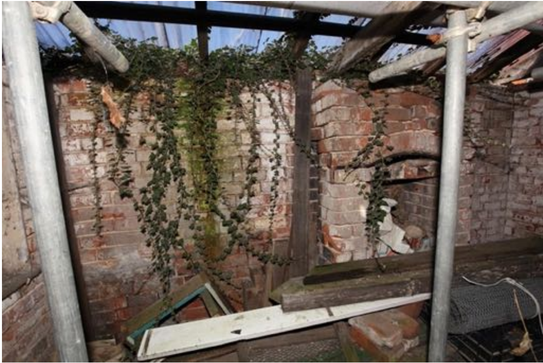
Illus. 11. The fireplace in the rear (northern) internal wall of the lean-to 'garden room' behind no. 24, which evidently operated as a wash house (G3). There is no evidence of a bread oven and the chimney has been lost. In its current form this structure was built between 1902 and 1924.
