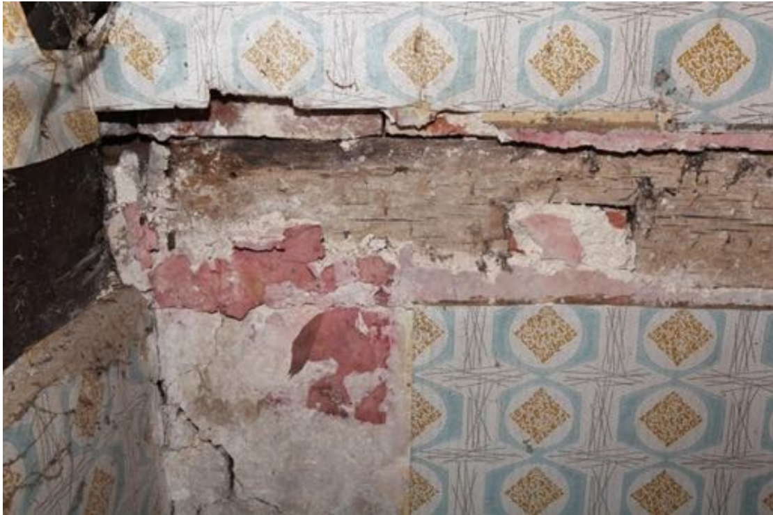
Illus. 49. A detail of the tie-beam in illustration 48 showing original or early red pigment and the notch that accommodates the brick rear wall of Lodge Cottage (F4). An identical notch is visible at the southern end of the same timber to the right in illustration 48, indicating the two cottages were built together. The tie-beam is tenoned to the roof-plates in a manner not seen prior to the 19 th century when such timbers were usually dovetailed.
