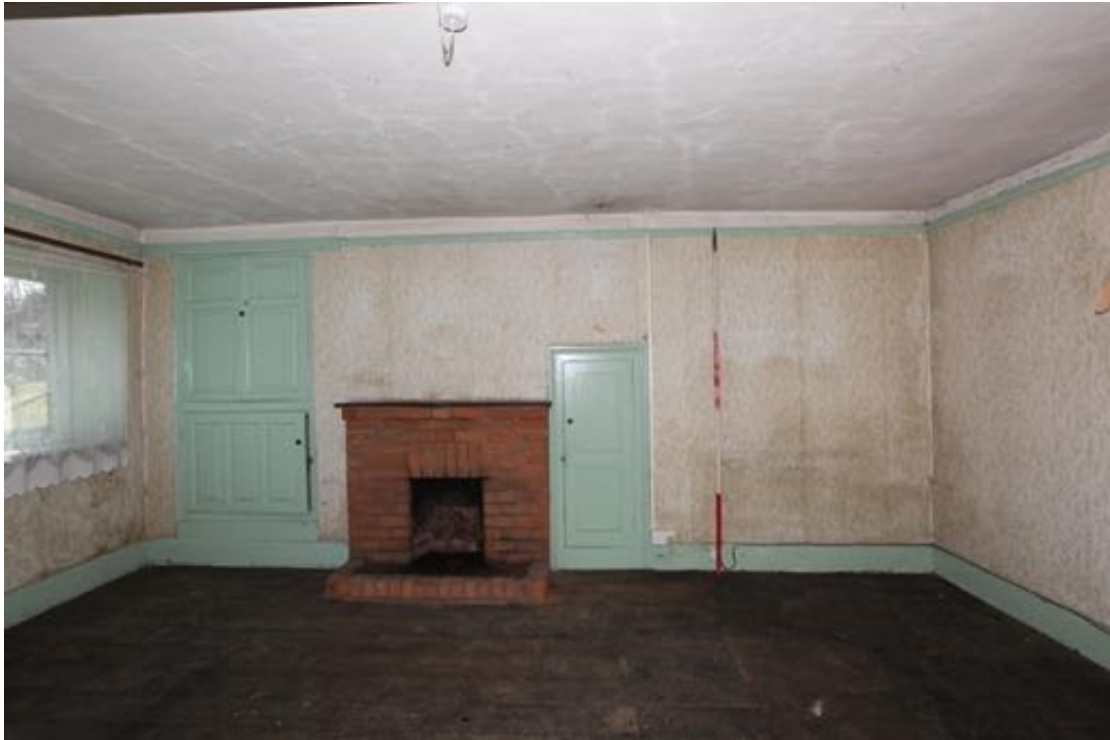
Illus. 37. The 20 th century brick fireplace in the western gable of the sitting room at no. 23 flanked by 19 th century cupboards with panelled doors (G5). The fireplace and right-hand cupboard occupy the position of a wider 19 th century fireplace.
