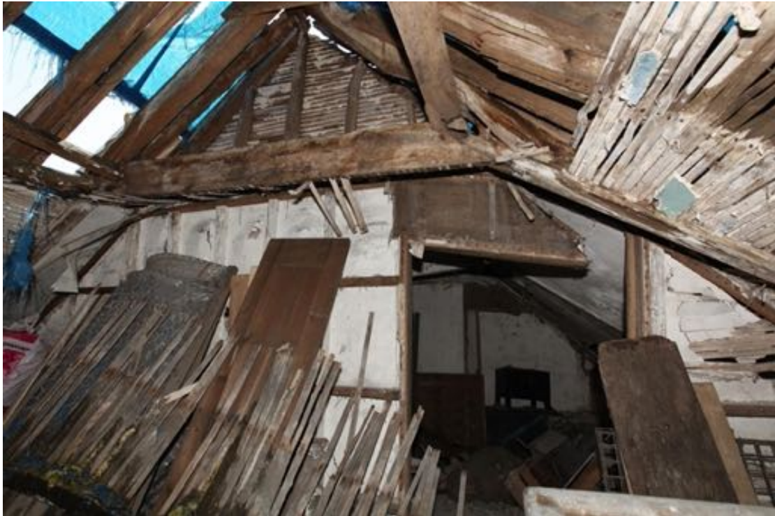
Illus. 29. The upper storey of no. 24 from the stair landing to the east (F2) showing the lath-and-plaster partition of the bedroom (F1) adjoining the clasped-purlin roof truss in the foreground. Much of the lower lath-and-plaster ceiling on the landing has collapsed.
