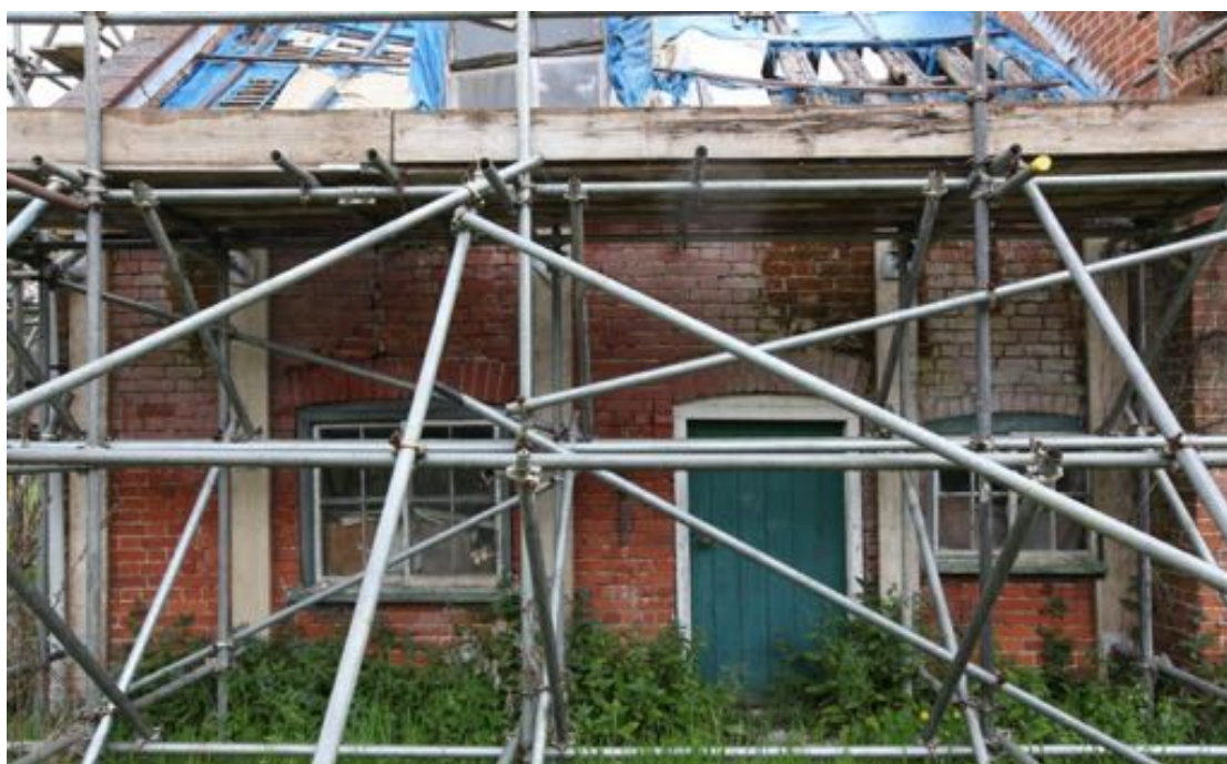
Illus. 2. The facade of no. 24 showing its entrance flanked by horizontal sash windows identical to those of no. 23. The segmental arches differ from the flat-topped arches of no. 23, indicating a slightly later date of construction, and the window on the right appears to be an early insertion as its arch consists of headers rather than stretchers. The Mock Tudor roof dormer is identical to those of no. 23 (see figure 10).
