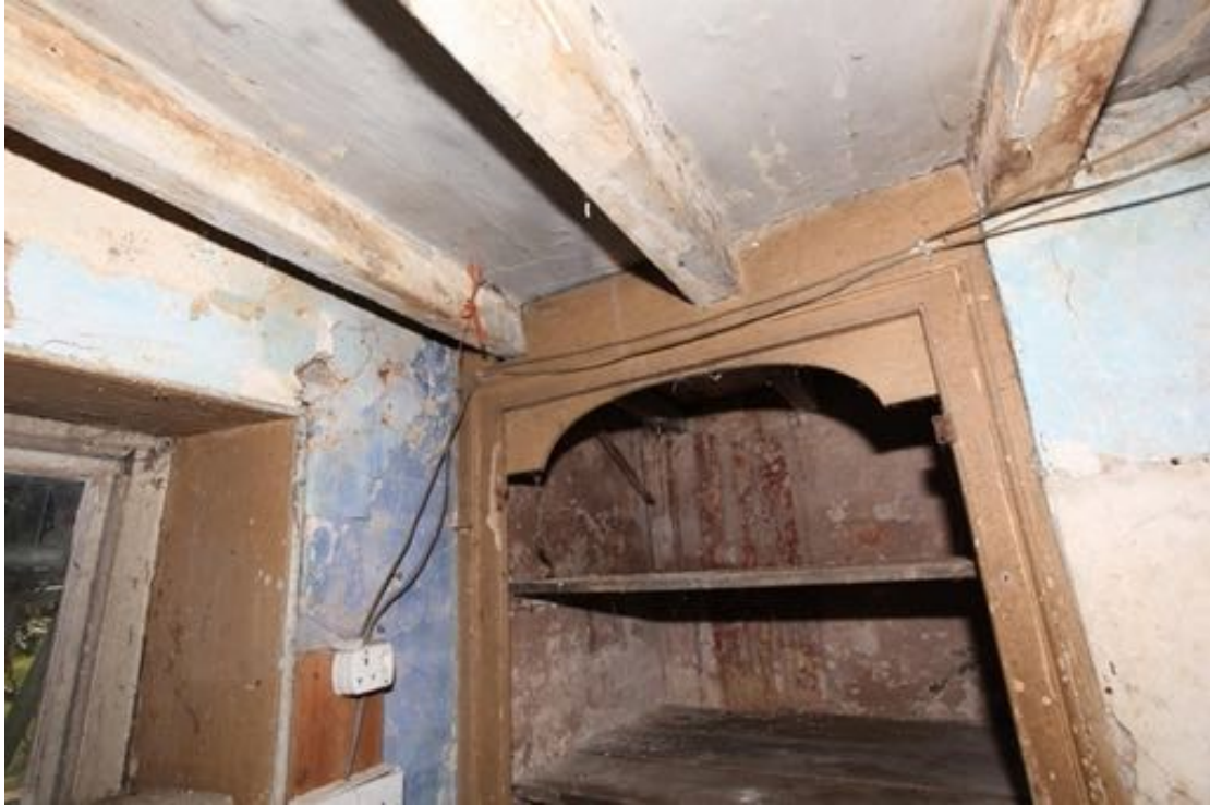
Illus. 21. A detail of the cupboard to the south of the western fireplace in the sitting room at no. 24 showing the hinges of its missing doors (G1).
