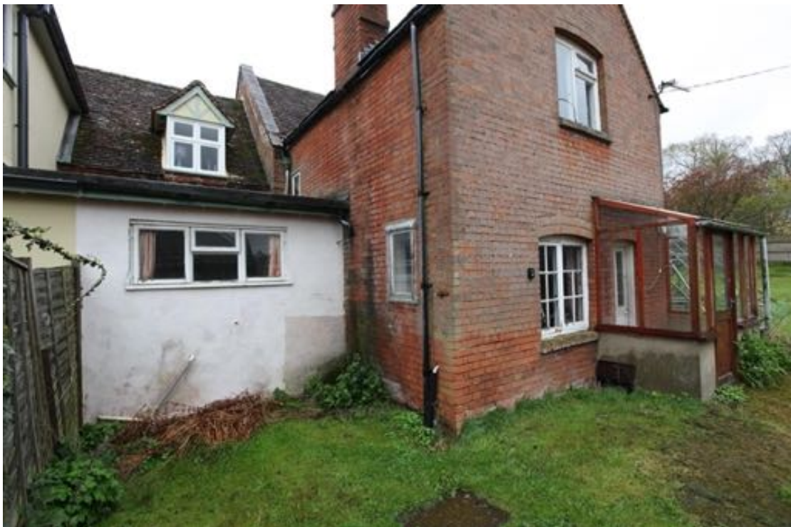
Illus. 8. The building from the north-east showing the large early-20 th century two-storied extension of no 23 added between 1902 and 1924 with the flat-roofed extension behind Lodge Cottage that contains its modern kitchen (G9) to the left. The modern rear glazed entrance porch preserves the scar of a smaller, earlier porch with a pitched roof.
