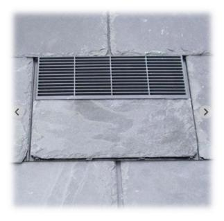
As one of the most versatile natural slate ventilators available on the market today, this Nature Vent will coordinate perfectly with any slate by easily using a piece of the same slate, cutting on site and fitting it into the bottom section.
