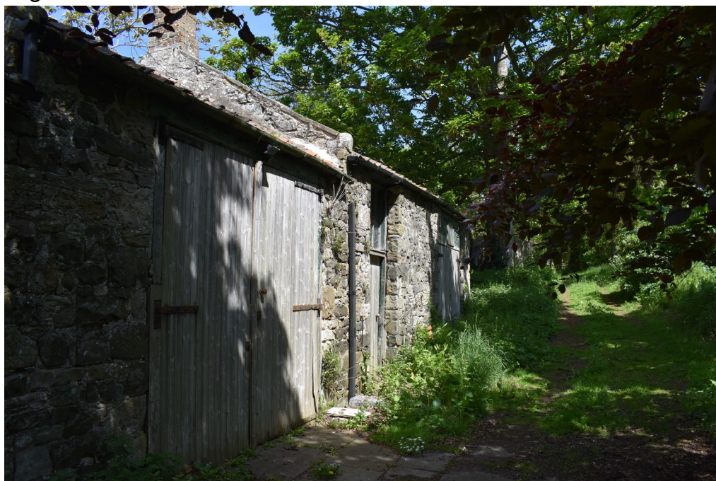
Access track connecting to the Embleton Tower driveway
