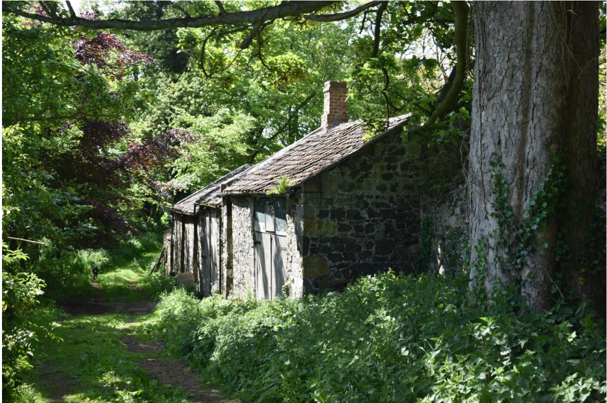
Outbuilding looking along the southern elevation
