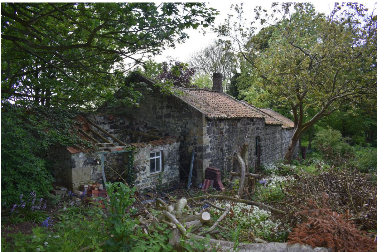
Outbuilding looking along the northern elevation
