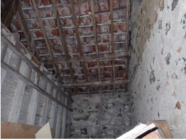
Pantiles with torching
