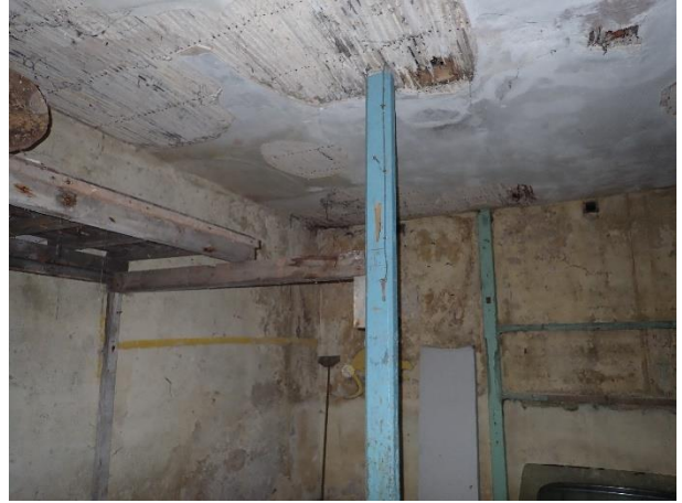
Latt and plastered section, propped.
