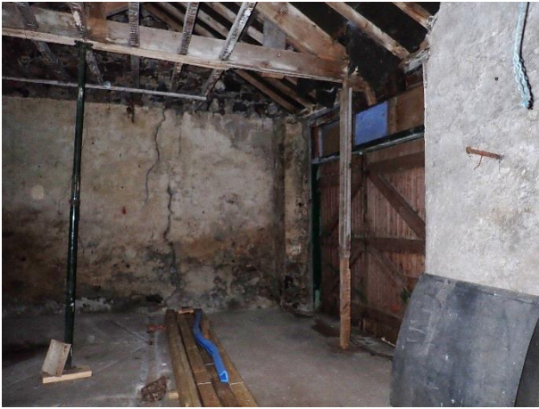
Northern section interior.
