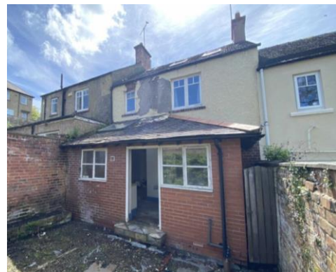
North elevation with existing ground floor extension.
