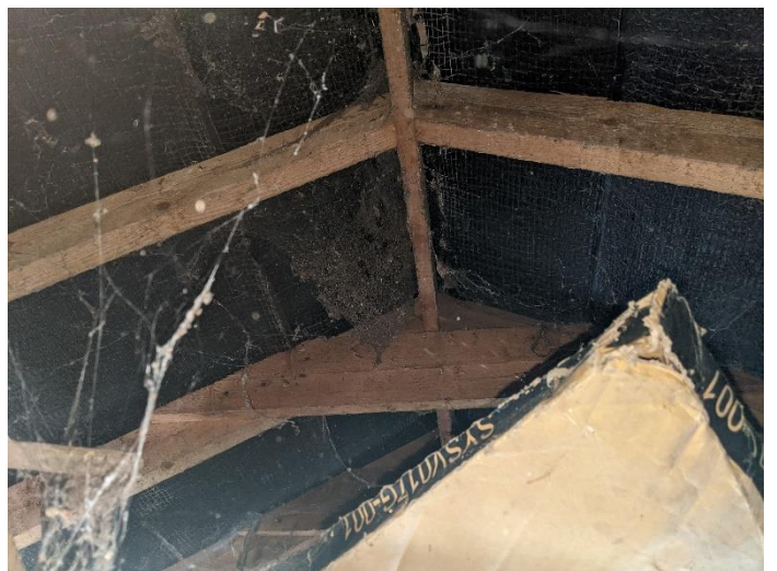
Photo 6 Felt roof – very cobwebby with no droppings internally
