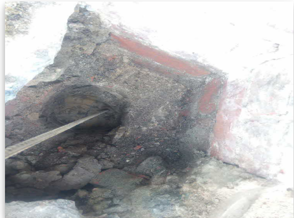
Fig 1.2: Trial Hole 1 Footing
