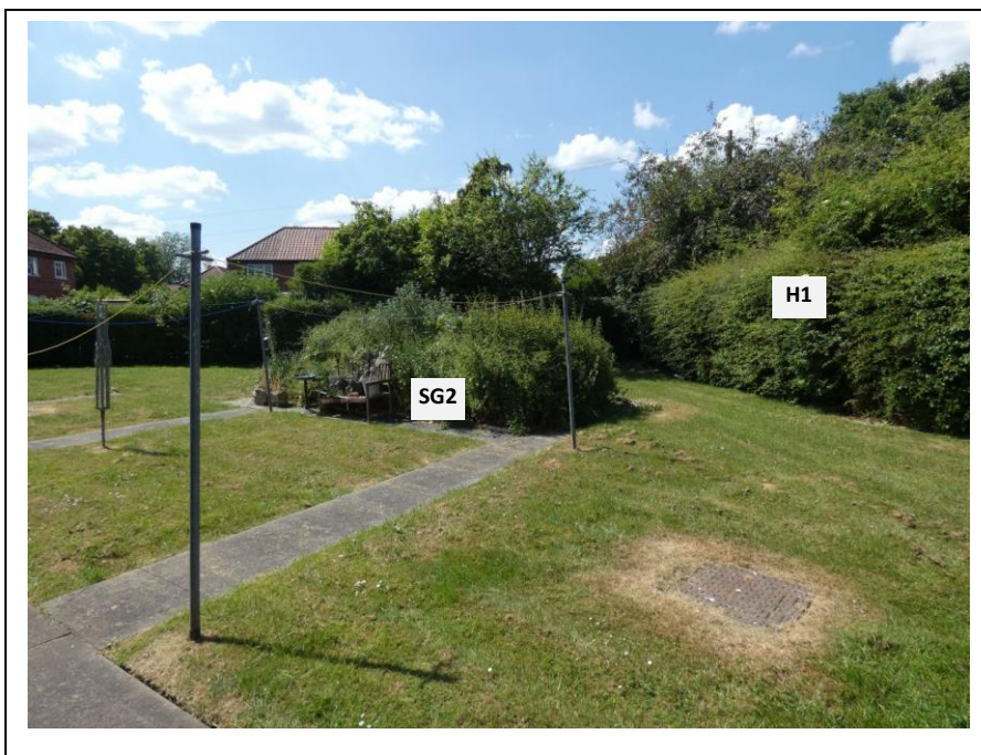
View of rear
