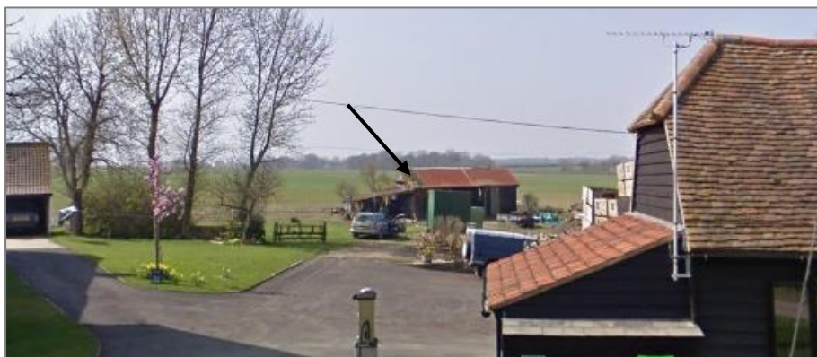
Figure 3 – Building prior to storm
