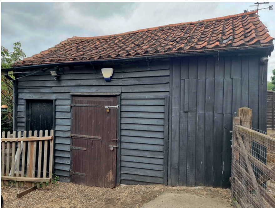
Side view of the Shed
