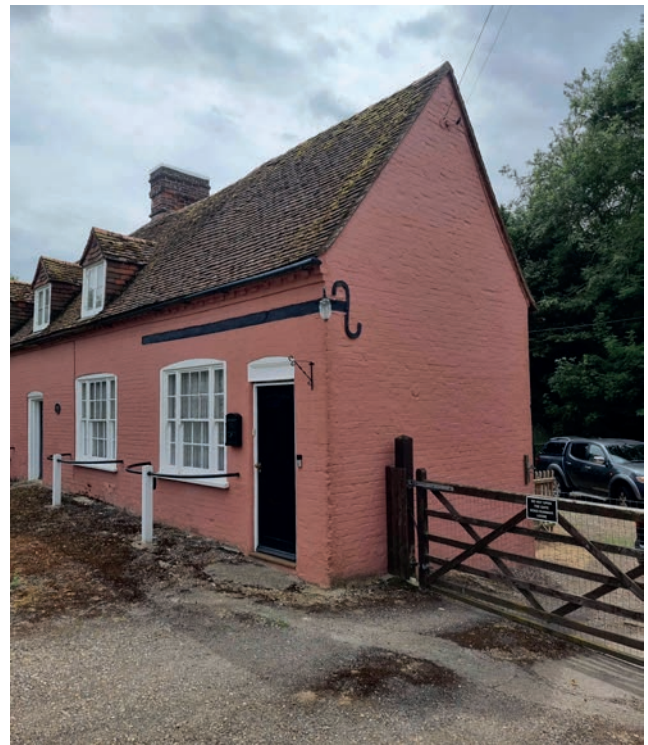
Front side view of Spread Eagle House
