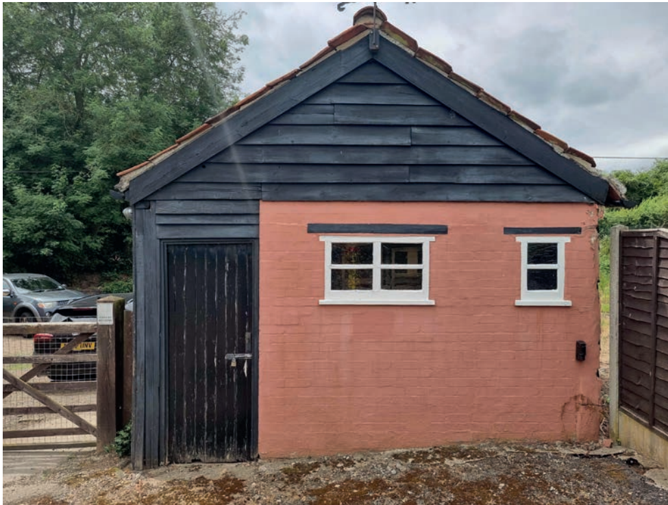
Front view of the Shed - which is behind tall hedging
