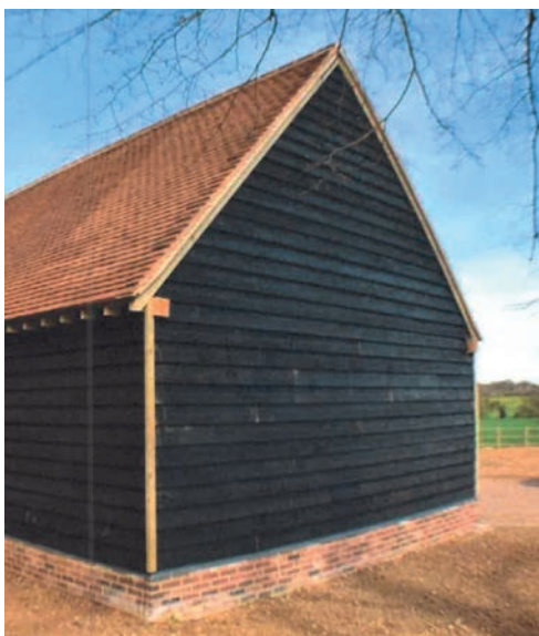
Example of exposed rafter feet, black weatherboards and brick plinth.
