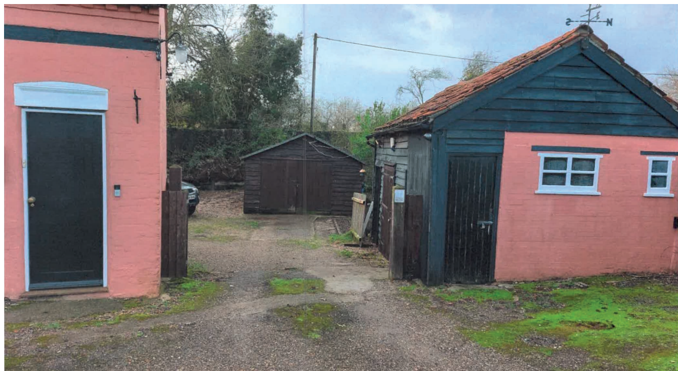
Front view of Spread Eagle House entrance showing existing garage behind the Shed.
