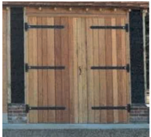
Timber boarded doors and strap hinges painted black
