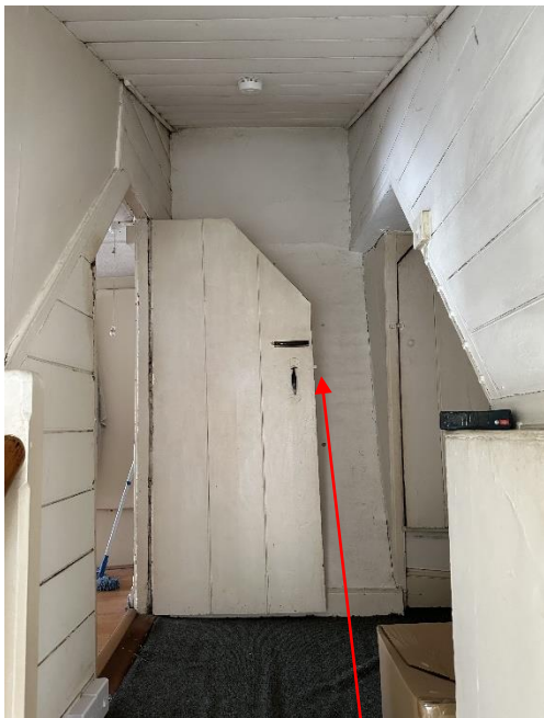
Top of 2 nd floor landing area.
