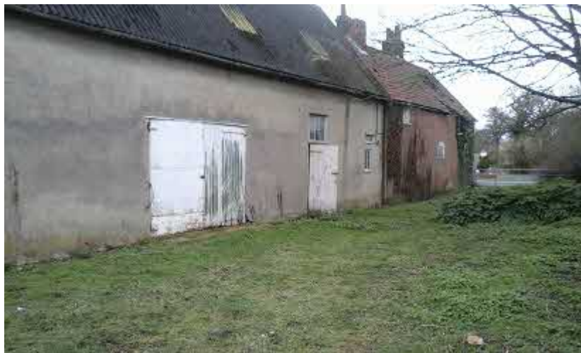
Tn 2. Traditional barn-rendered exterior; also showing rear of Tn 1 and area Tn 15.
