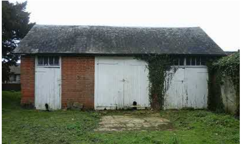
Tn 5. Double Garage and storage building.
