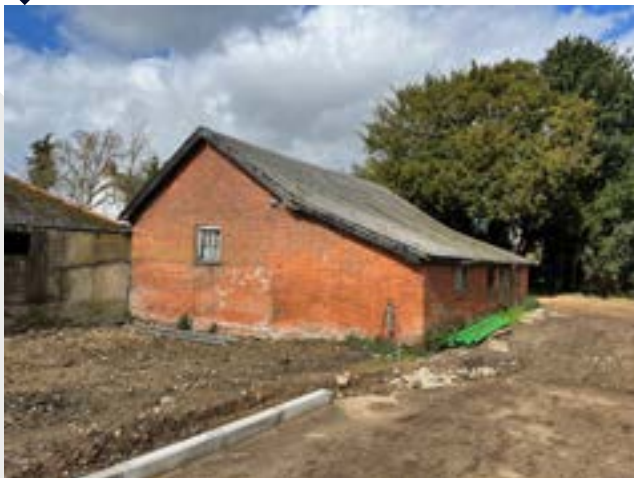
▼ Southern side of the workshop
