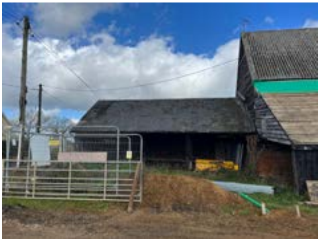
3 Bay cart lodge on the west end of Essex Barn
