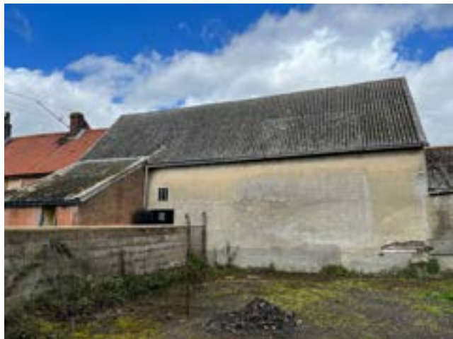
▲ Front of the Stable Barn. External dividing wall to be removed.
