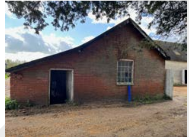
▲ Northern side of the workshop
