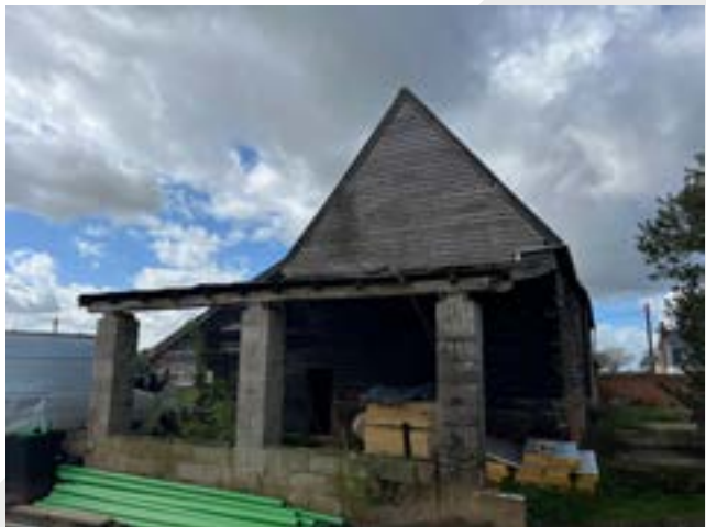
East gable end view
