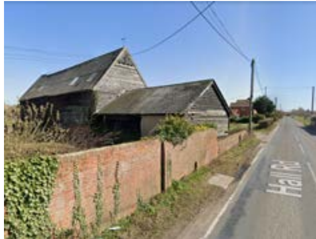
▲ Google Street View image of existing brick boundary wall to be set further back to accommodate visibility splay
