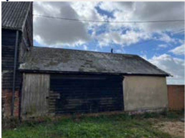
Rear access to the 3 bay cart lodge
