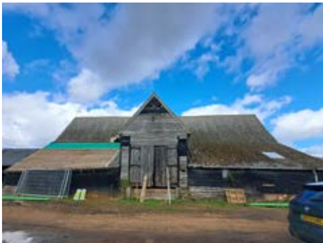
Front of the Essex Barn
