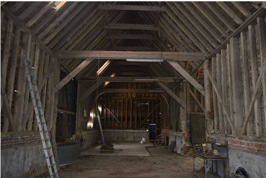
Figure 10: North-East internal elevation of the barn.
