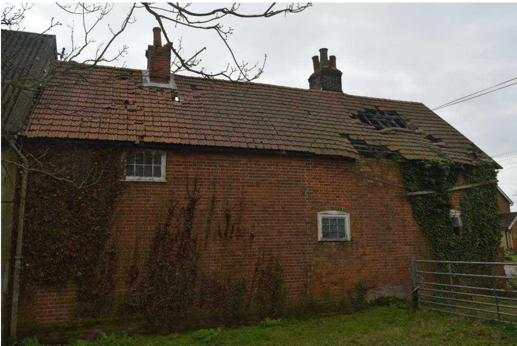
Figure 16: North-West (rear) elevation of the workers cottages.
