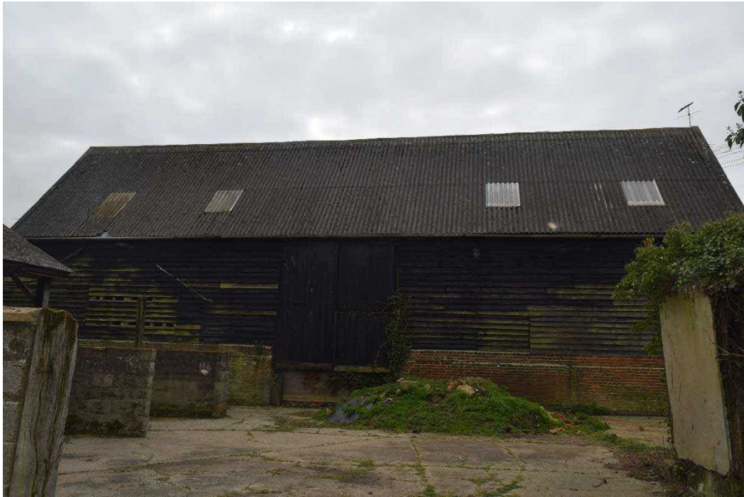
Figure 8: North-West elevation of the barn.
