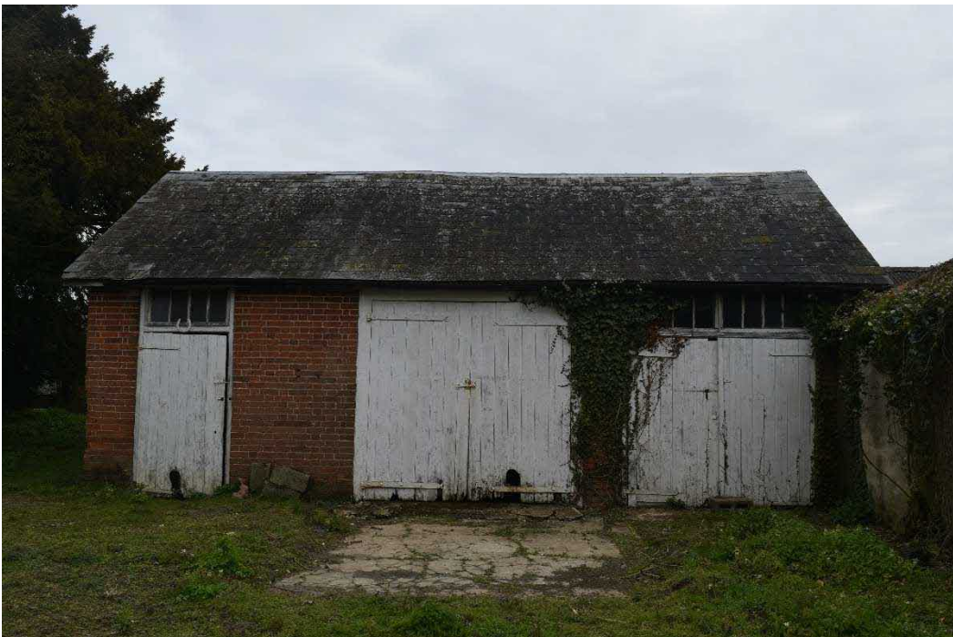
Figure 30: South-West elevation of the Workshop.
