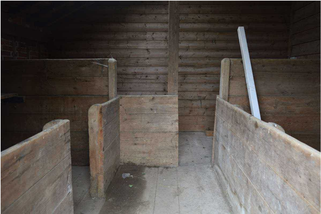
Figure 13: Granary outshot on the South-East elevation of the barn.
