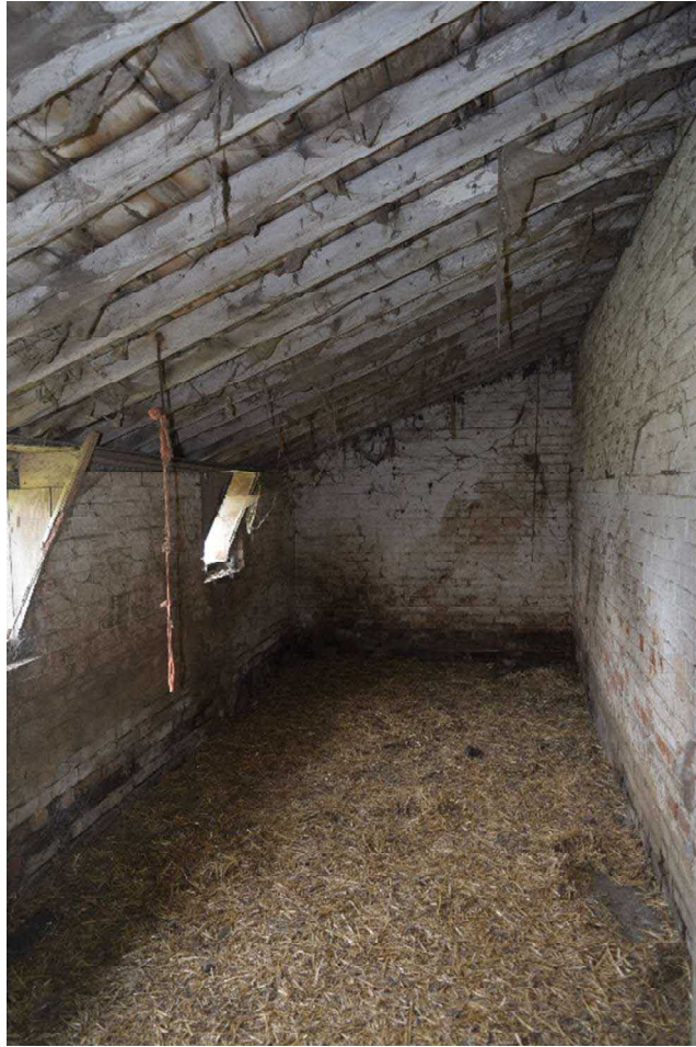
Figure 35: Animal shelter to the rear of the garage.
