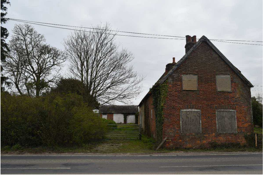
Figure 17: South-West gable end of the workers cottages.
