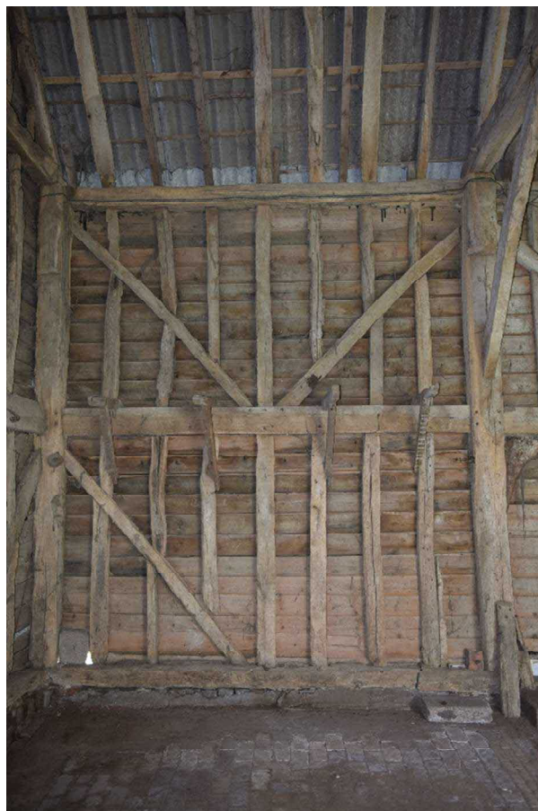
Figure 24: Wall framing assemblage.
