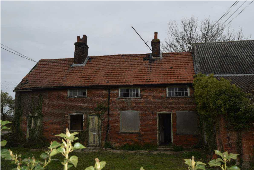
Figure 15: South-East (front) elevation of the workers cottages.
