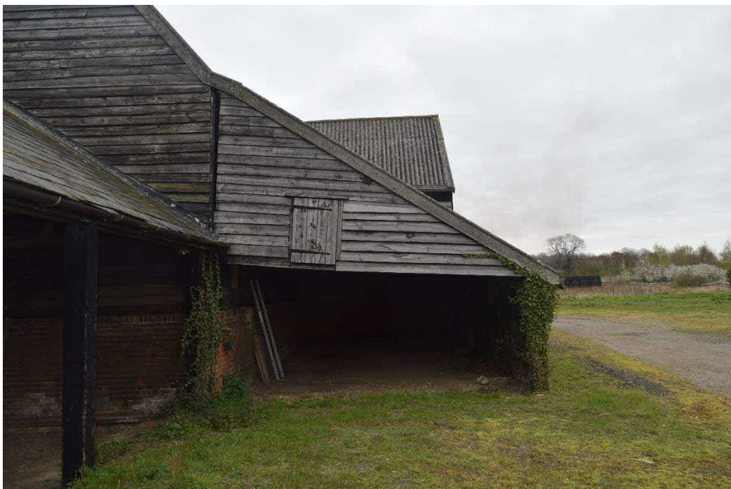
Figure 12: Carshed outshot on the South-East elevation of the barn.
