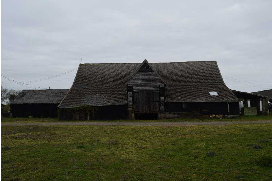
Figure 6: South-East elevation of the barn.
