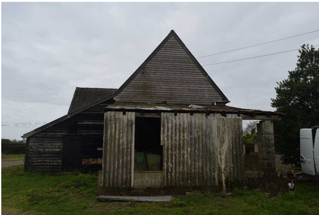
Figure 7: North-East elevation of the barn.
