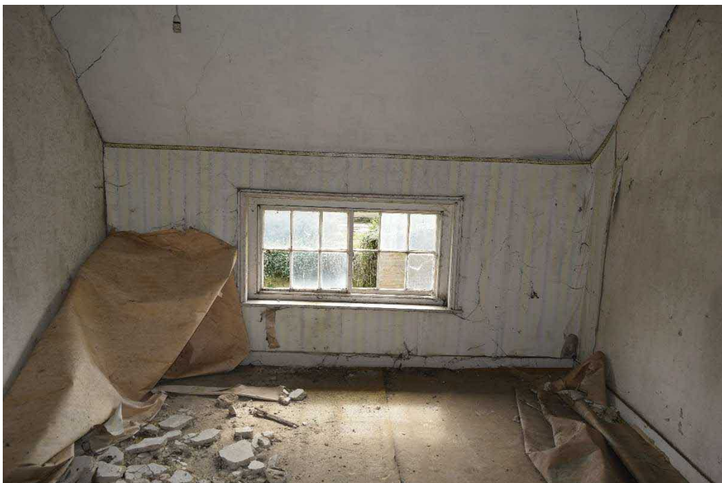
Figure 20: First Floor bedroom over cottage 2 (kitchen).
