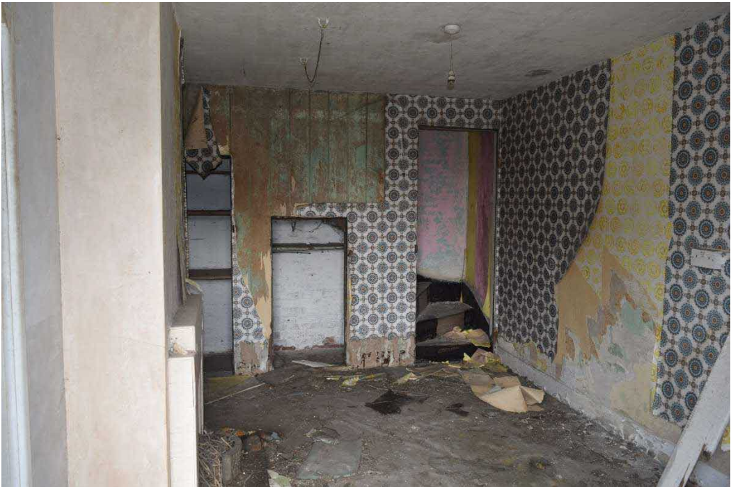
Figure 18: Ground Floor of cottage 2 (kitchen).
