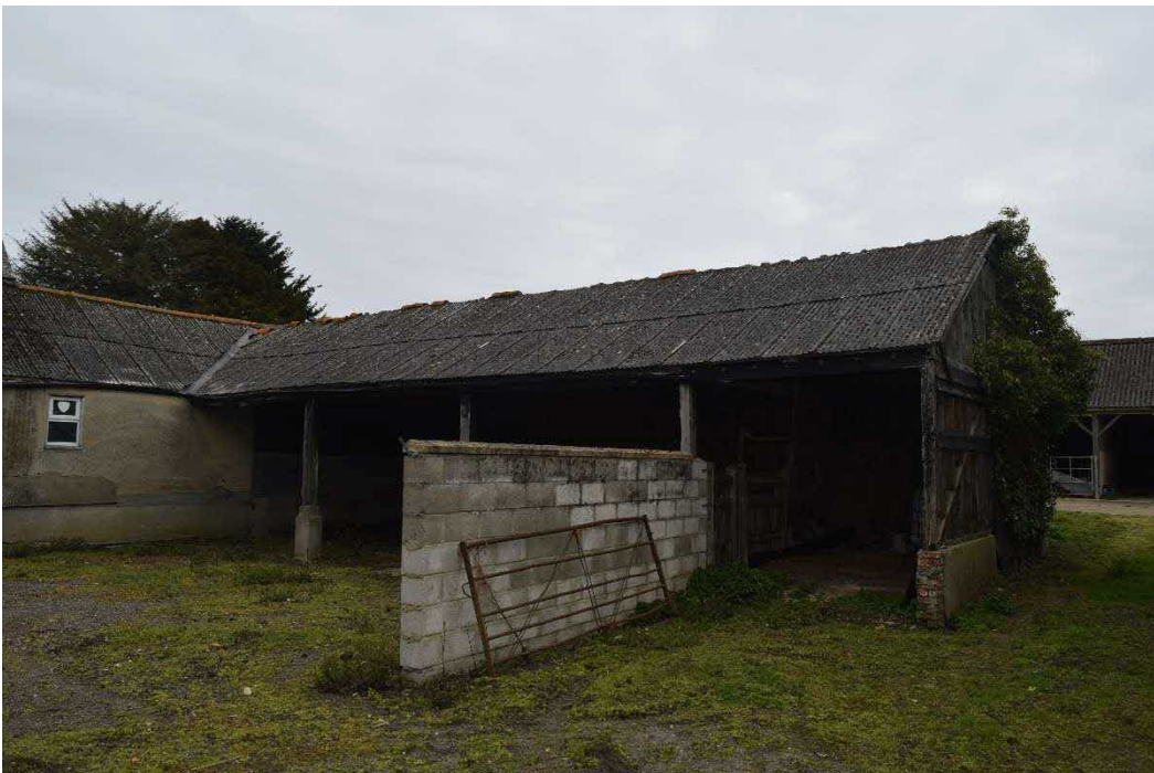
Figure 27: C19/C20 Open fronted shelter shed partly rebuilt.
