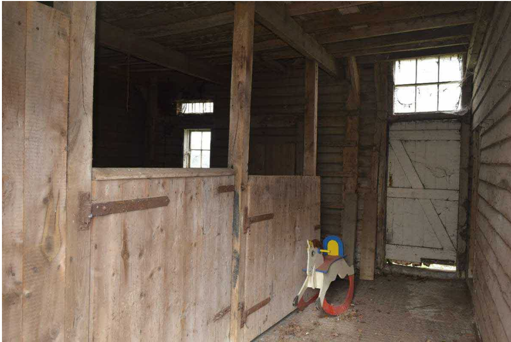
Figure 25: Stables at the South-West end of the barn with hayloft over.
