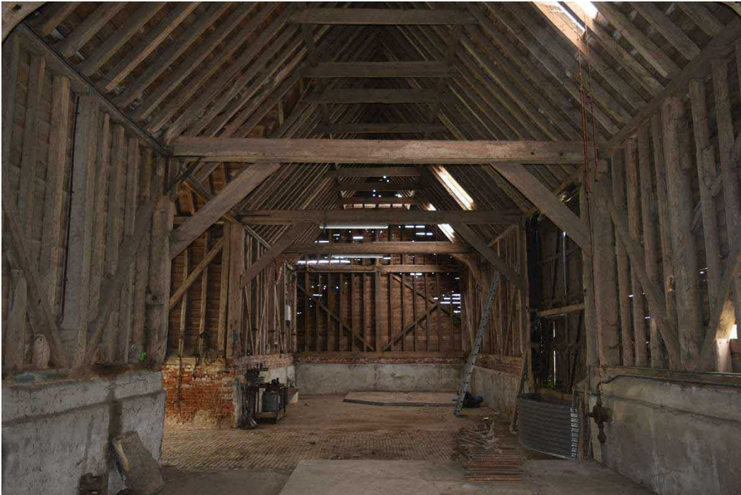
Figure 9: South-West internal elevation of the barn.
