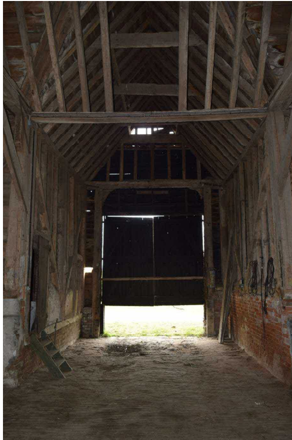
Figure 11: Internal view of the midstrey on the South-East elevation of the barn.
