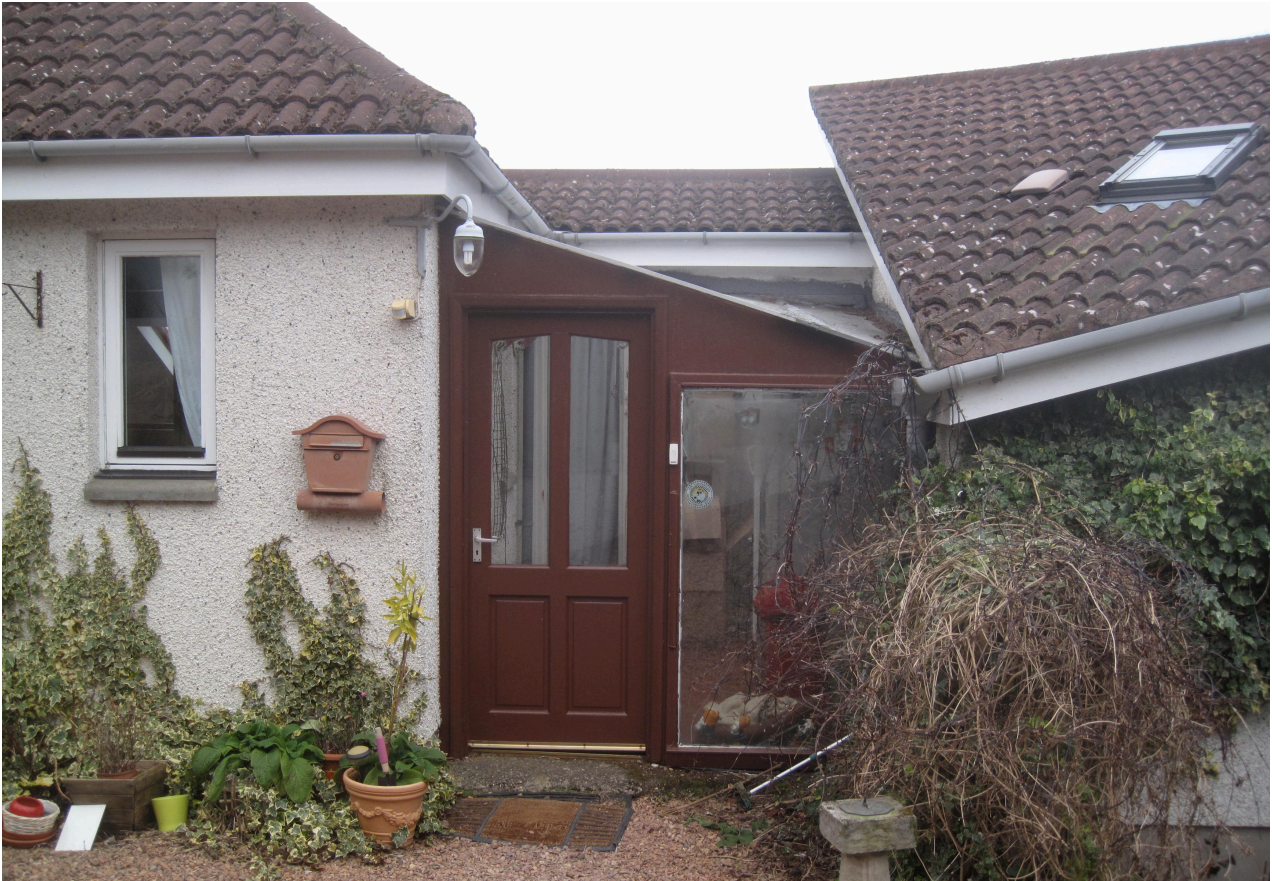
Access to Self Contained Annex
