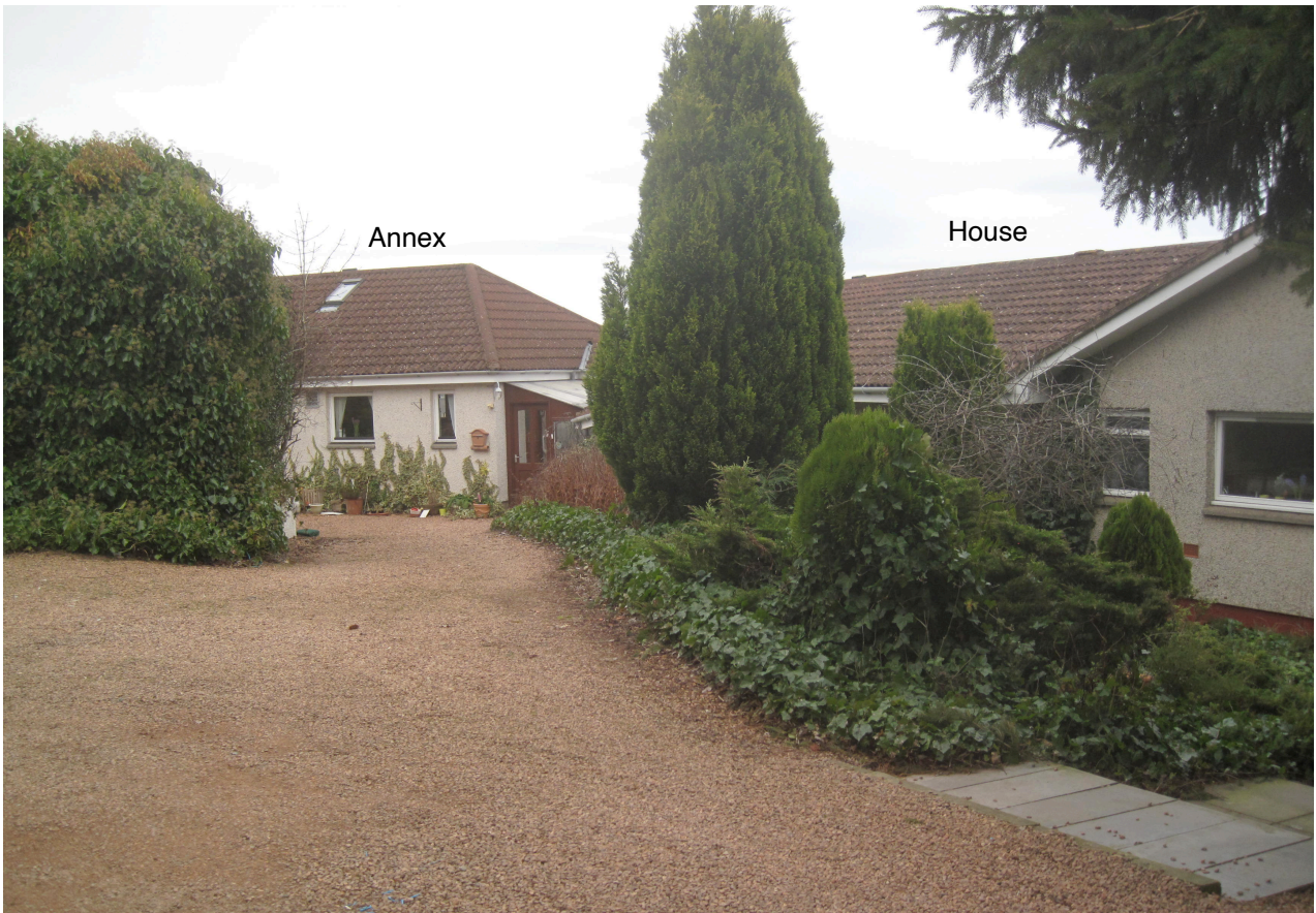
View northwards from driveway towards self contained annex
