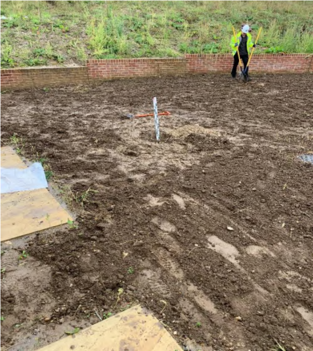
Photographs 1-2 , taken on the 01 st September 2023 showing examples of hand dug trial pits and the nature of the subsoil and topsoil within the soft landscaping of plot 86 (back garden).
