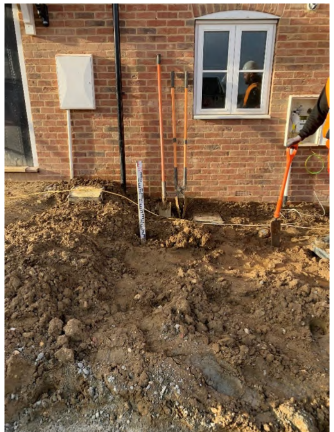
Photographs 12-15 , taken on the 13 th January 2023 showing examples of hand dug trial pits and the nature of the subsoil and topsoil within the soft landscaping of plot 114 (representative of plots 112-117).
