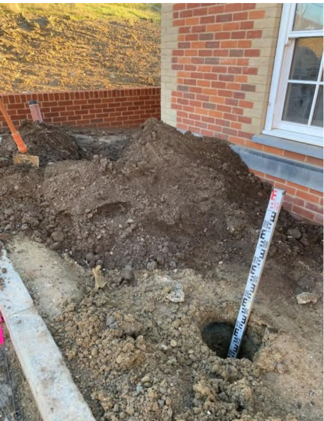
Photographs 9-12 , taken on the 08 th December 2022 showing examples of hand dug trial pits and the nature of the subsoil and topsoil within the soft landscaping of plot 68 (representative of plots 118, 119 and 67-69).
