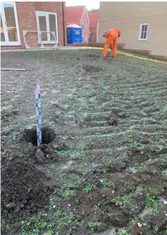
Photographs 5-8 , taken on the 08 th December 2022 showing examples of hand dug trial pits and the nature of the subsoil and topsoil within the soft landscaping of plot 67 (representative of plots 118, 119 and 67-69).
