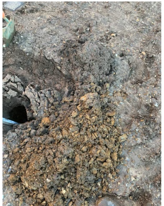
Photographs 9-12 , taken on the 08 th December 2022 showing examples of hand dug trial pits and the nature of the subsoil and topsoil within the soft landscaping of plot 68 (representative of plots 118, 119 and 67-69).
