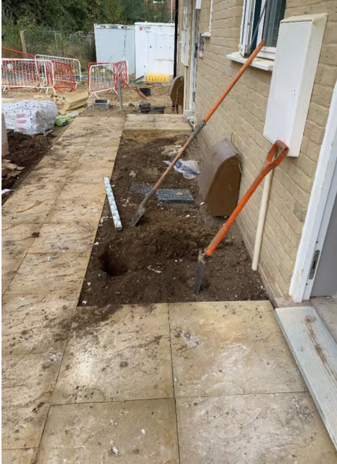
Photographs 9-10 , taken on the 28 th September 2022 showing the topsoil thickness (200mm) within the front gardens of plot 122 (representative of plots 121-123).
