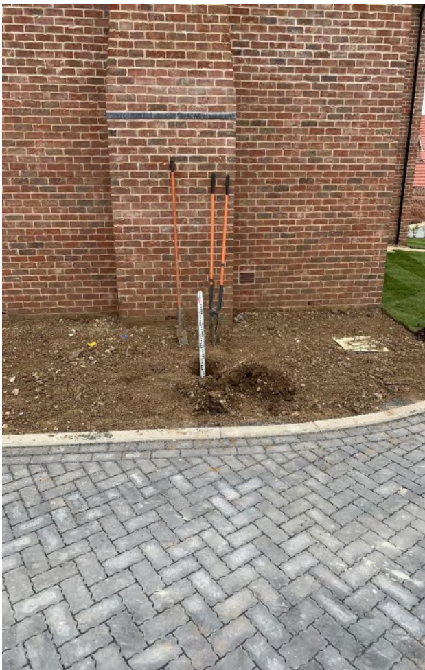
Photographs 1-4 , taken on the 19 th May 2023 showing examples of hand dug trial pits and the nature of the subsoil and topsoil within the soft landscaping of plot 77 (back and front garden).
