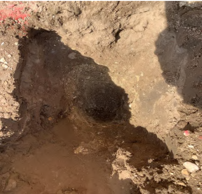
Photographs 5-8 , taken on the 09 th August 2022 showing examples of hand dug trial pits and the nature of the subsoil and topsoil within the soft landscaping of plot 198 (representative of plots 197-199 & 200-203).
