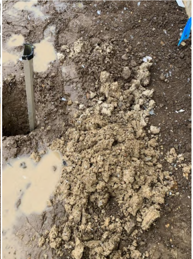
Photographs 8-11 , taken on the 10 th March 2023 showing examples of hand dug trial pits and the nature of the subsoil and topsoil within the soft landscaping of plot 74 (front garden).
