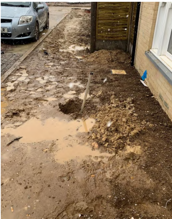
Photographs 8-11 , taken on the 10 th March 2023 showing examples of hand dug trial pits and the nature of the subsoil and topsoil within the soft landscaping of plot 74 (front garden).
