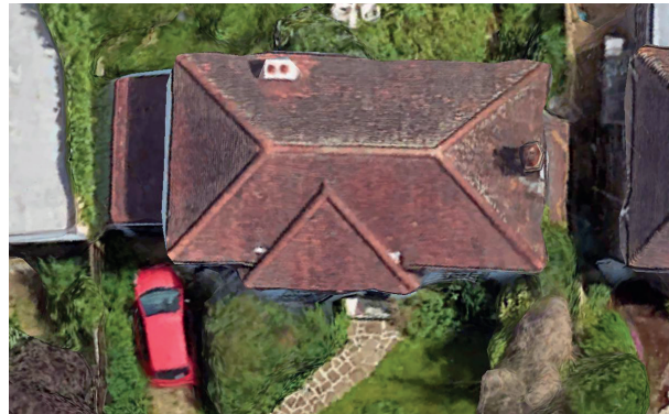
Aerial view of roof
