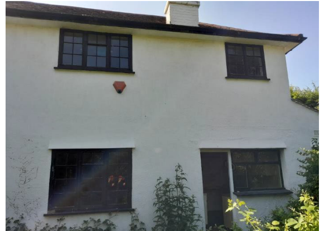
Figure 4. Central and south bay of the rear elevation
