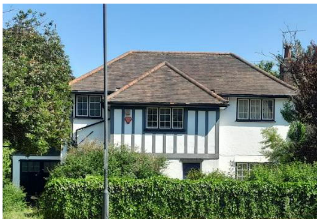
Figure 1. Front (west) elevation of the subject property.
