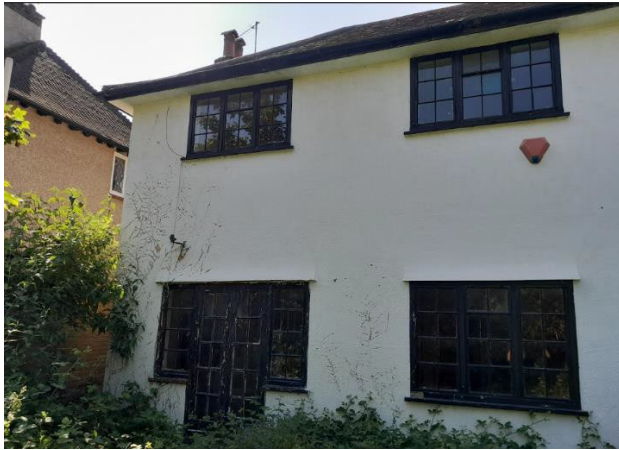
Figure 3. Central and north bay of the rear elevation.
