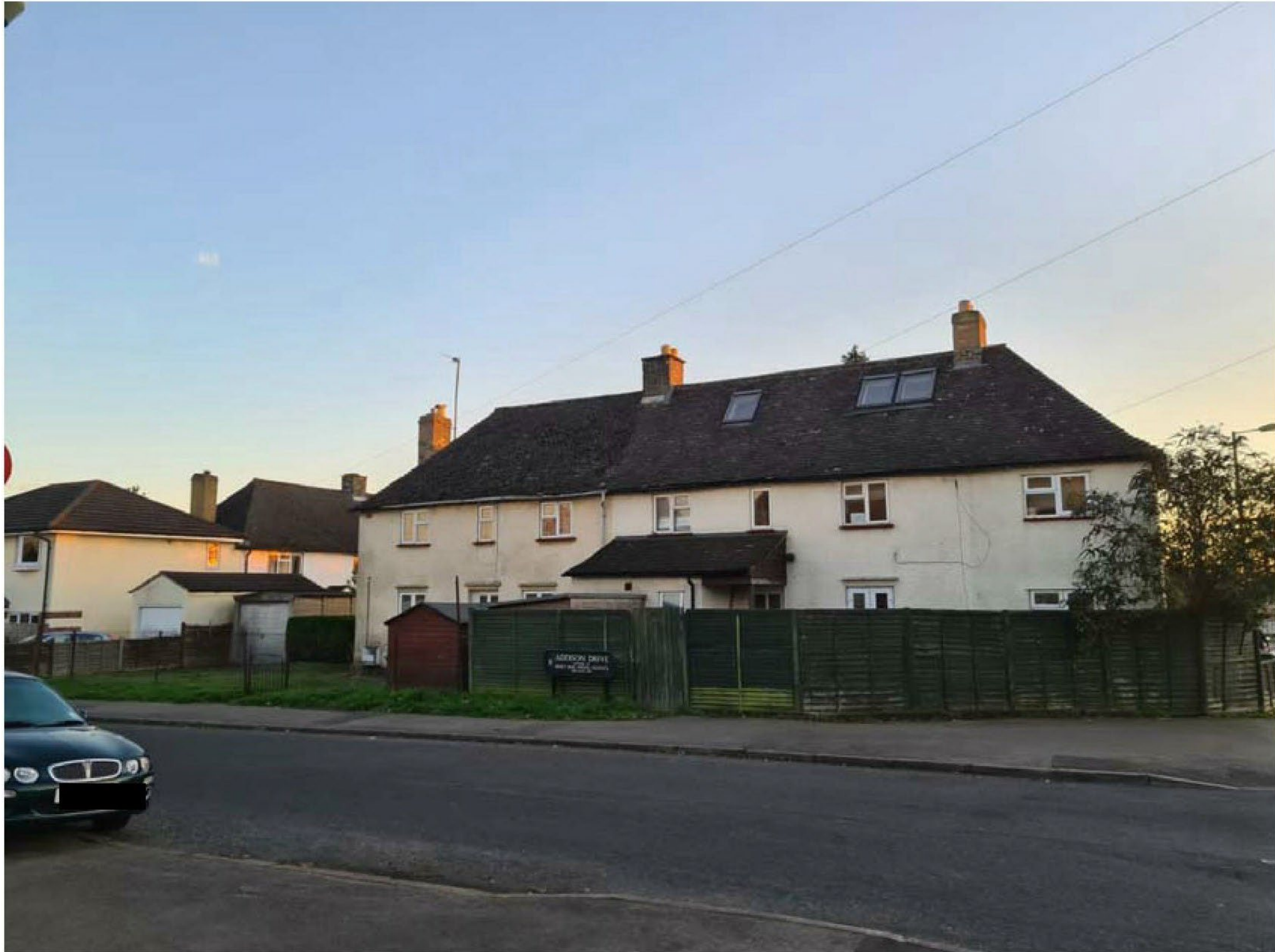
View of rear elevation from Addison Drive with No. 112 and side extension to right.
