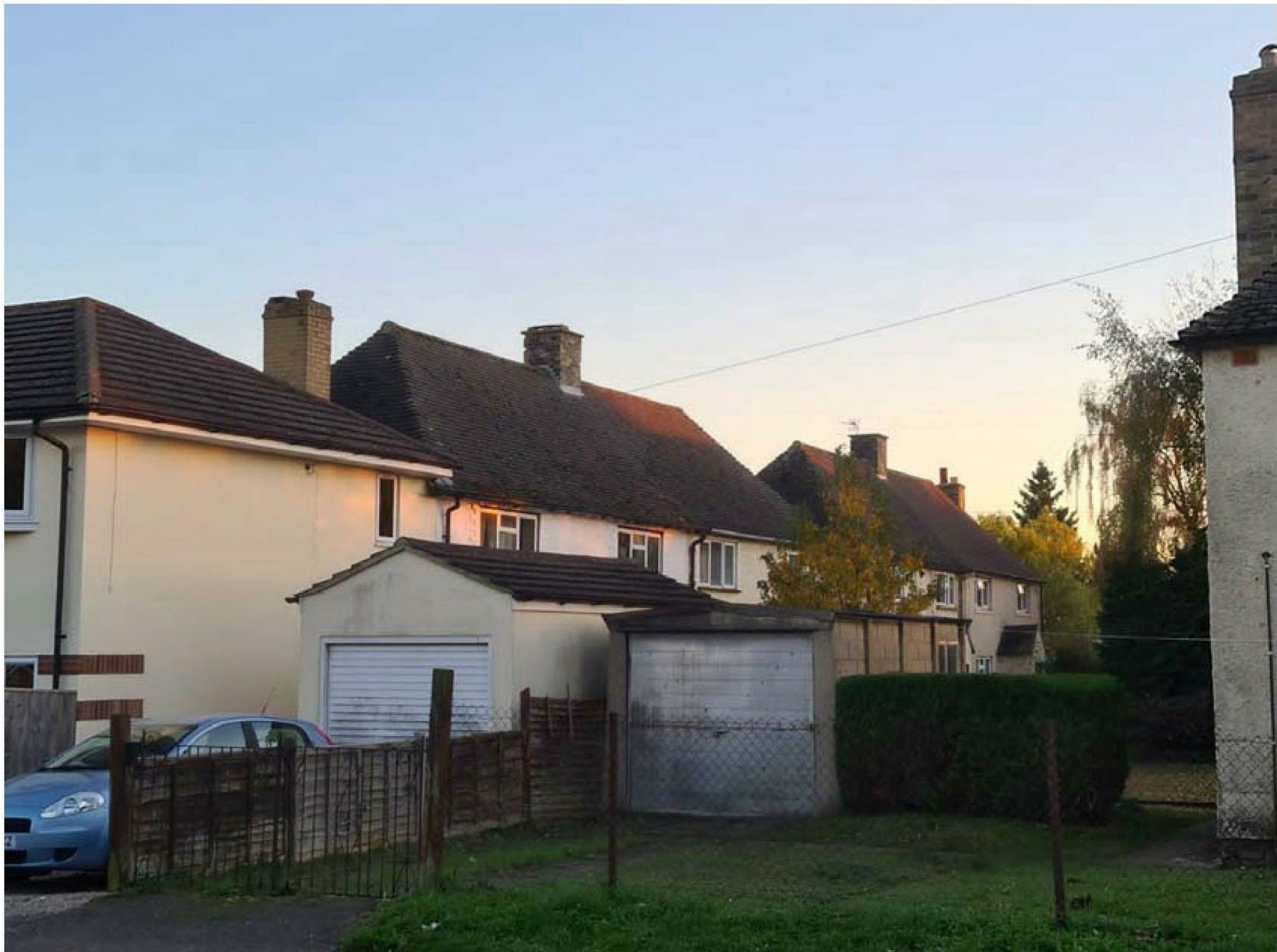
View of development plot to side of original dwelling with detached garage
